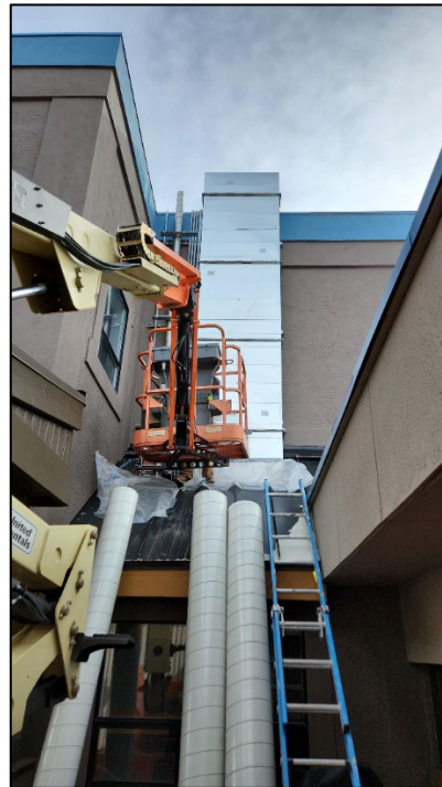
Installation of HVAC ductwork and conduit
