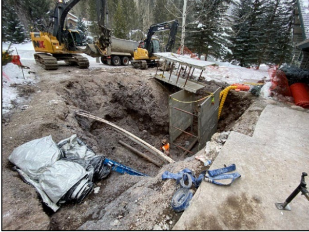
A deep and difficult excavation
