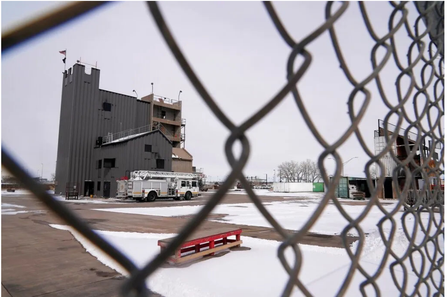
The Denver Fire Academy is visible through a fence from the road Thursday, Feb. 23, 2023, in Commerce City, Colo. Firefighting foam used here up until 2018 is suspected to be linked to the discovery of PFAS, or "forever chemicals" found in city's groundwater. (AP Photo/Brittany Peterson)
