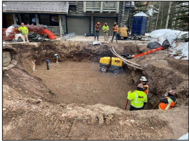
Backfilling after repairs
