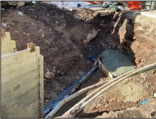
New pipe installation
