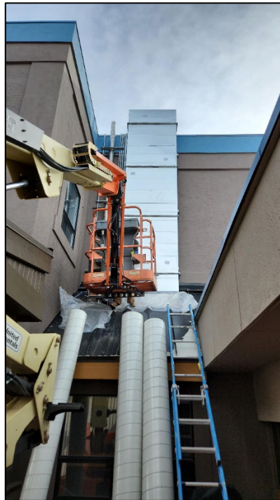
Installation of HVAC ductwork and conduit
