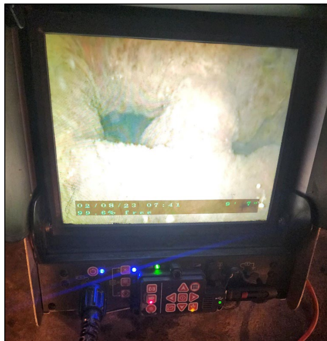
Submersible camera screenshot showing grate obstruction in secondary clarifier effluent pipe
