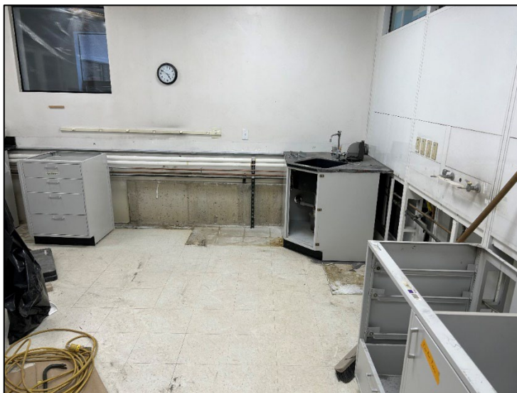
Counter and cabinet demolition in preparation for new fume hood
