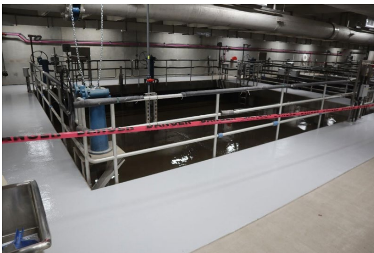
Progress of aeration basin floor coatings
