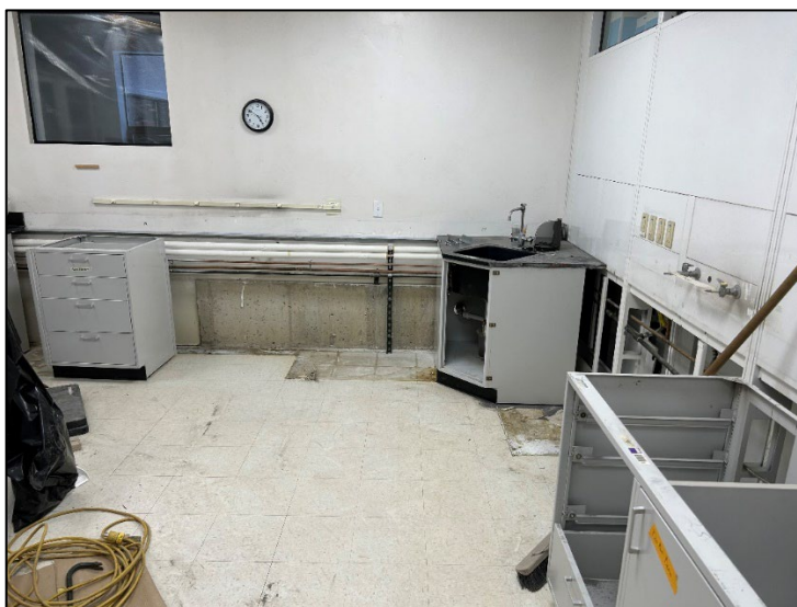
Counter and cabinet demolition in preparation for new fume hood
