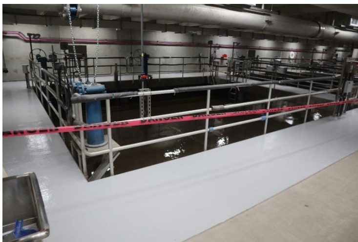
Progress of aeration basin floor coatings
