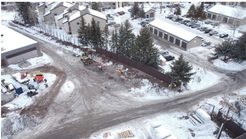
Aerial image of fence installation along western property boundary
