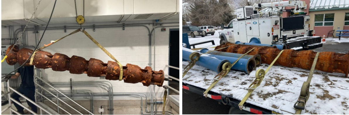
Finished water pump removal and preparation for transport
