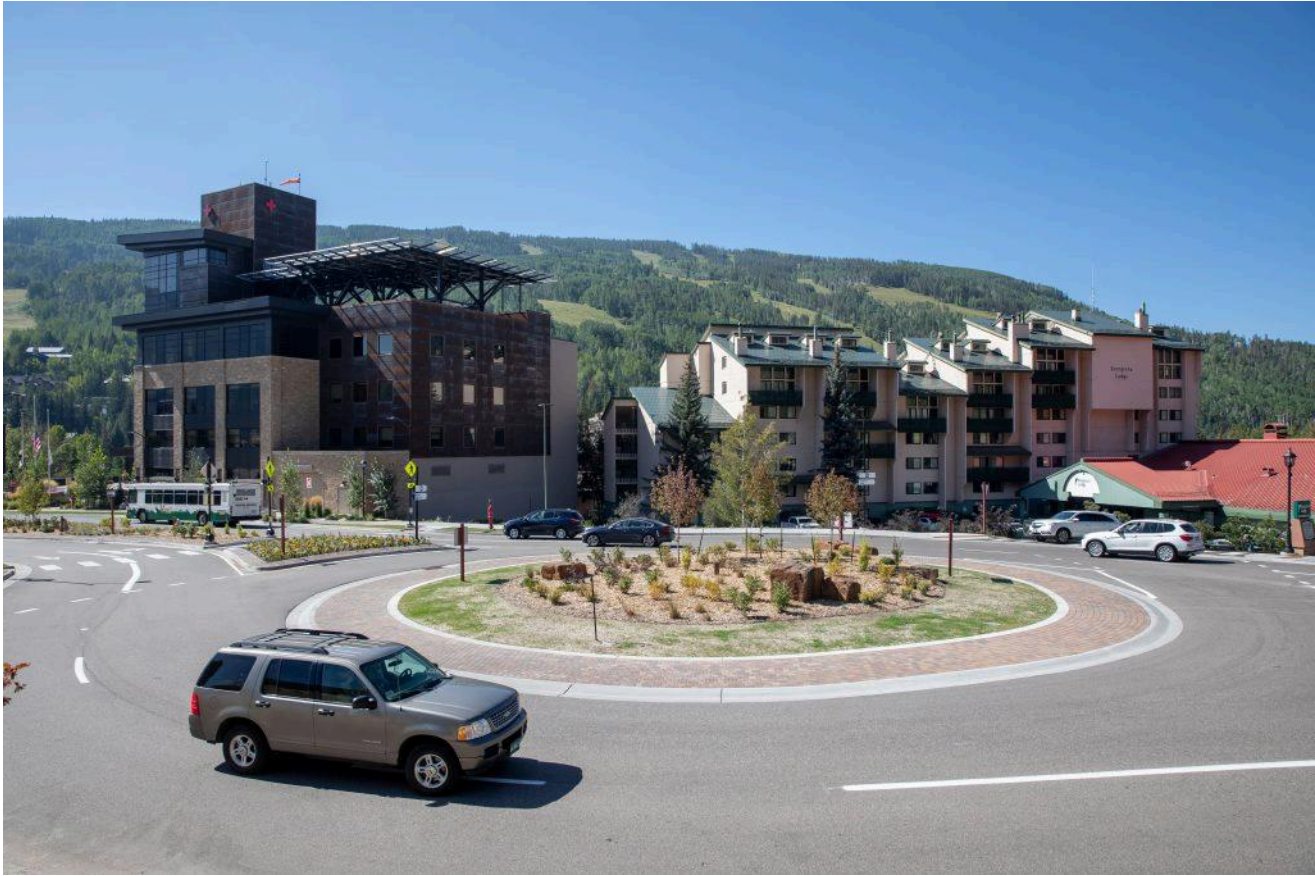
Vail's newest roundabout near Vail Health Hospital is an example of low-turf landscaping, which is part of the town's overall plan to reduce its water use. Town of Vail/Courtesy Photo
