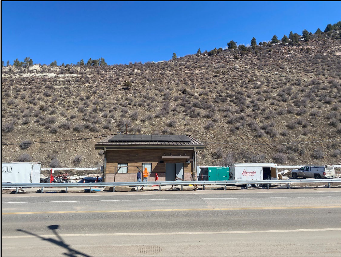
Exterior view of the lift station showing solar panels on roof
