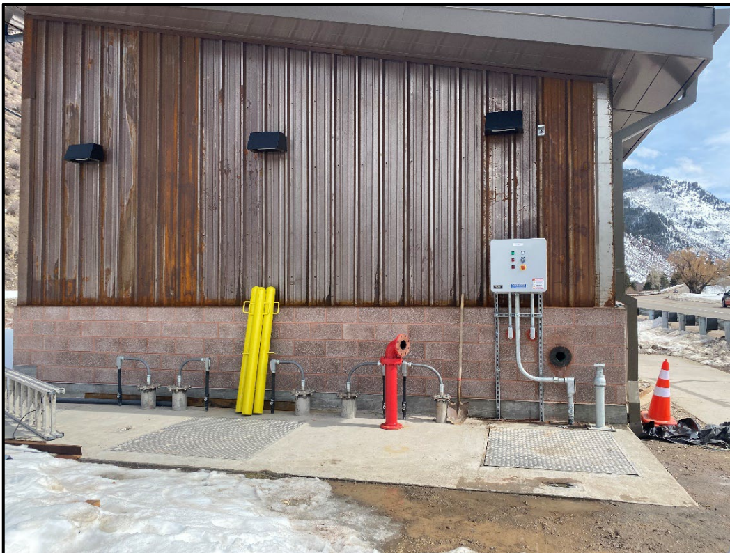
Wet well exterior on the west side of lift station
