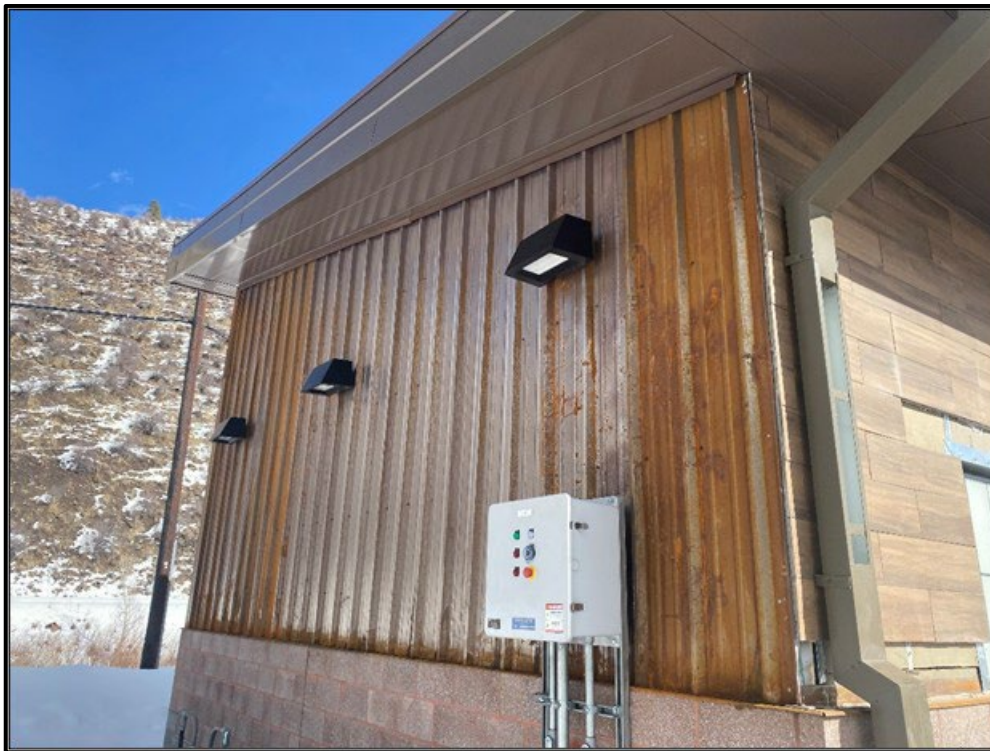
Exterior light fixture installation above the wet well
