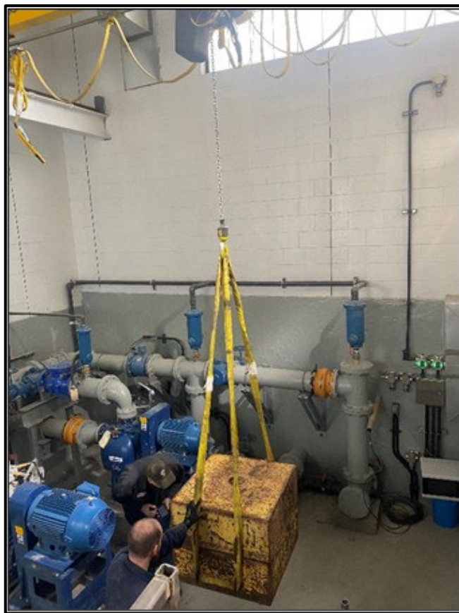
Load testing and start-up of the bridge crane
