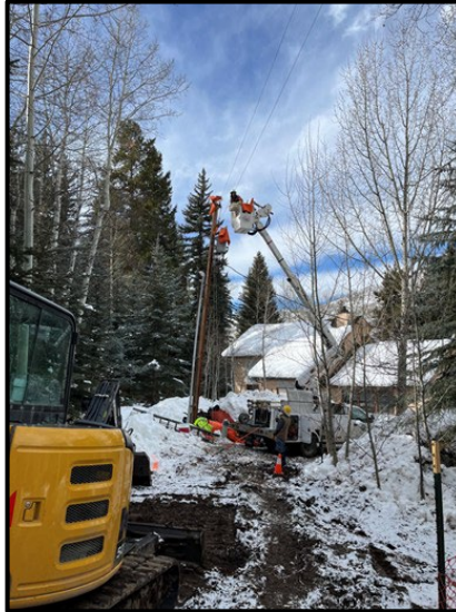
De-energizing power line
