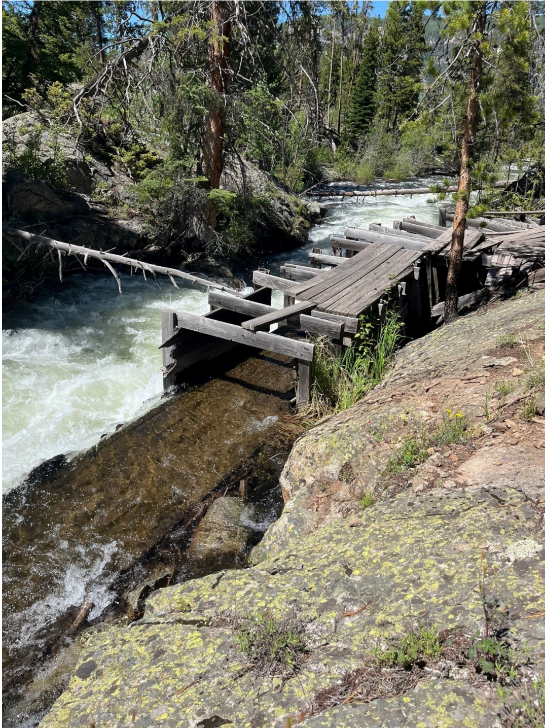
Attachment C: Photograph of Bolts Ditch intake and diversion structure
