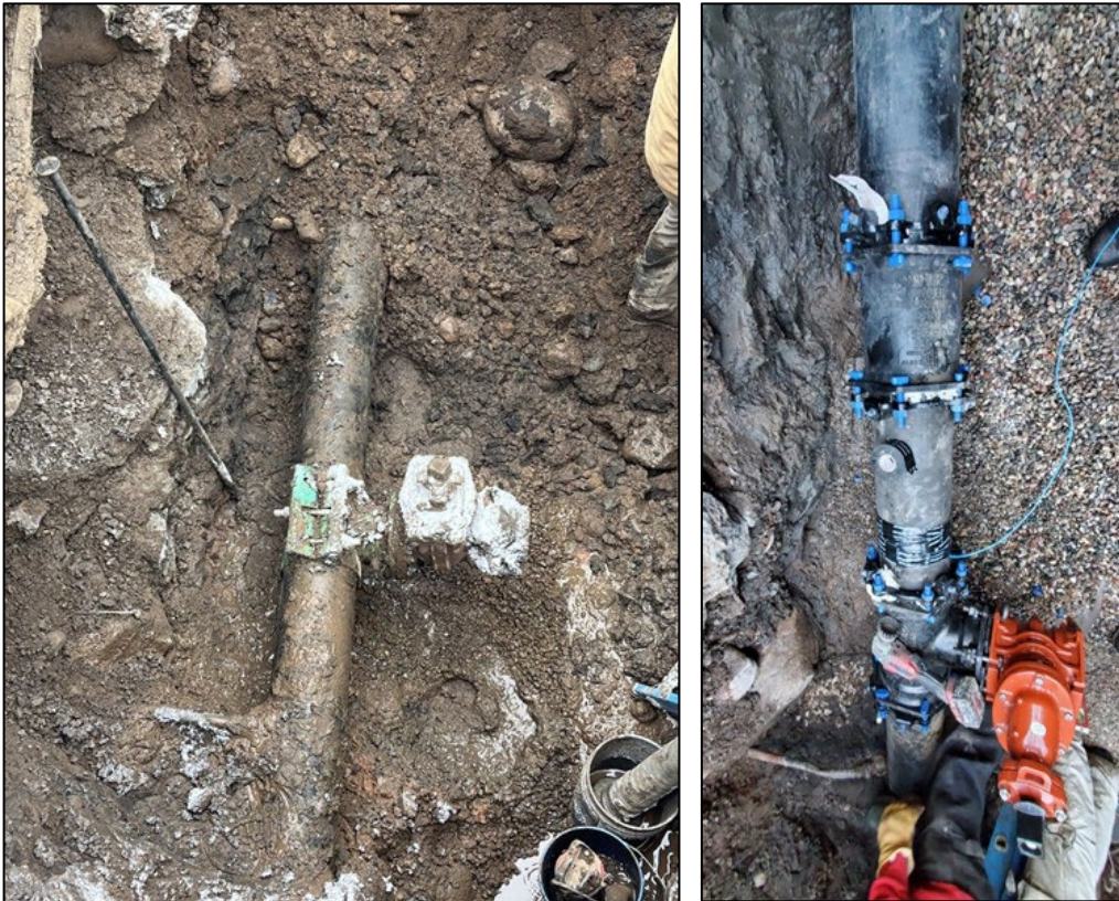
Valve and main replacement (before and after)
