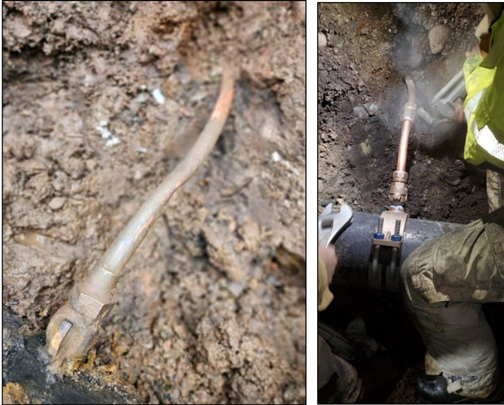
Damaged service pipe replacement (before and after)
