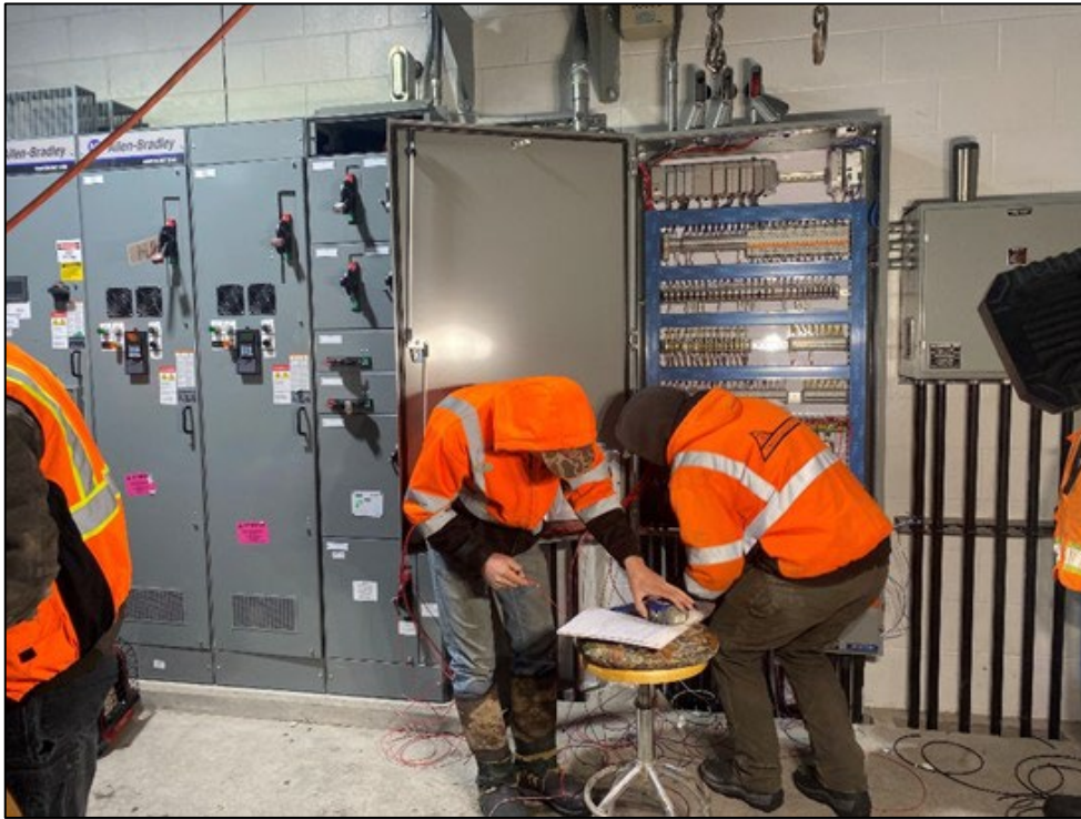
Interior electrical and control wire installation
