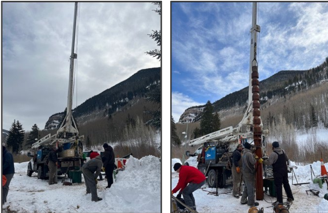
Well R7 motor installation
