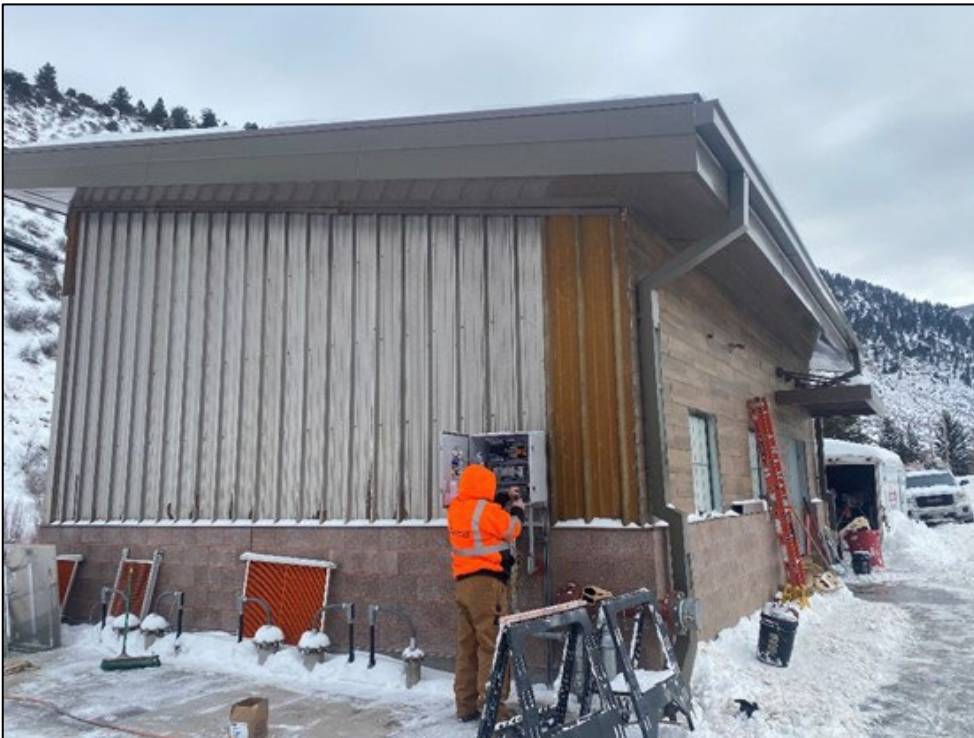
Exterior electrical and control wire installation
