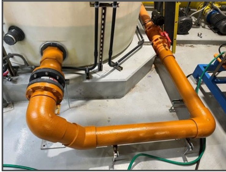
EDWF clean-in-place (CIP) pipe installation
