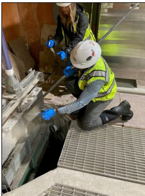
New UV system performance testing
