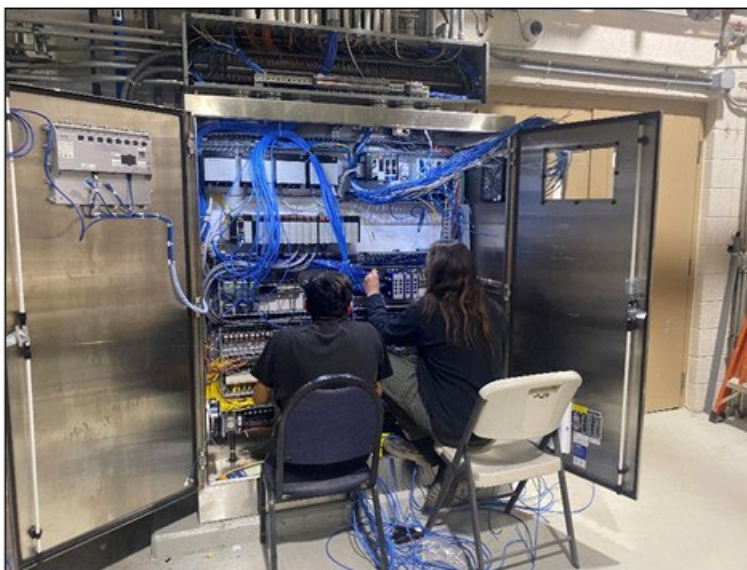
PLC #1 cable and wire installation
