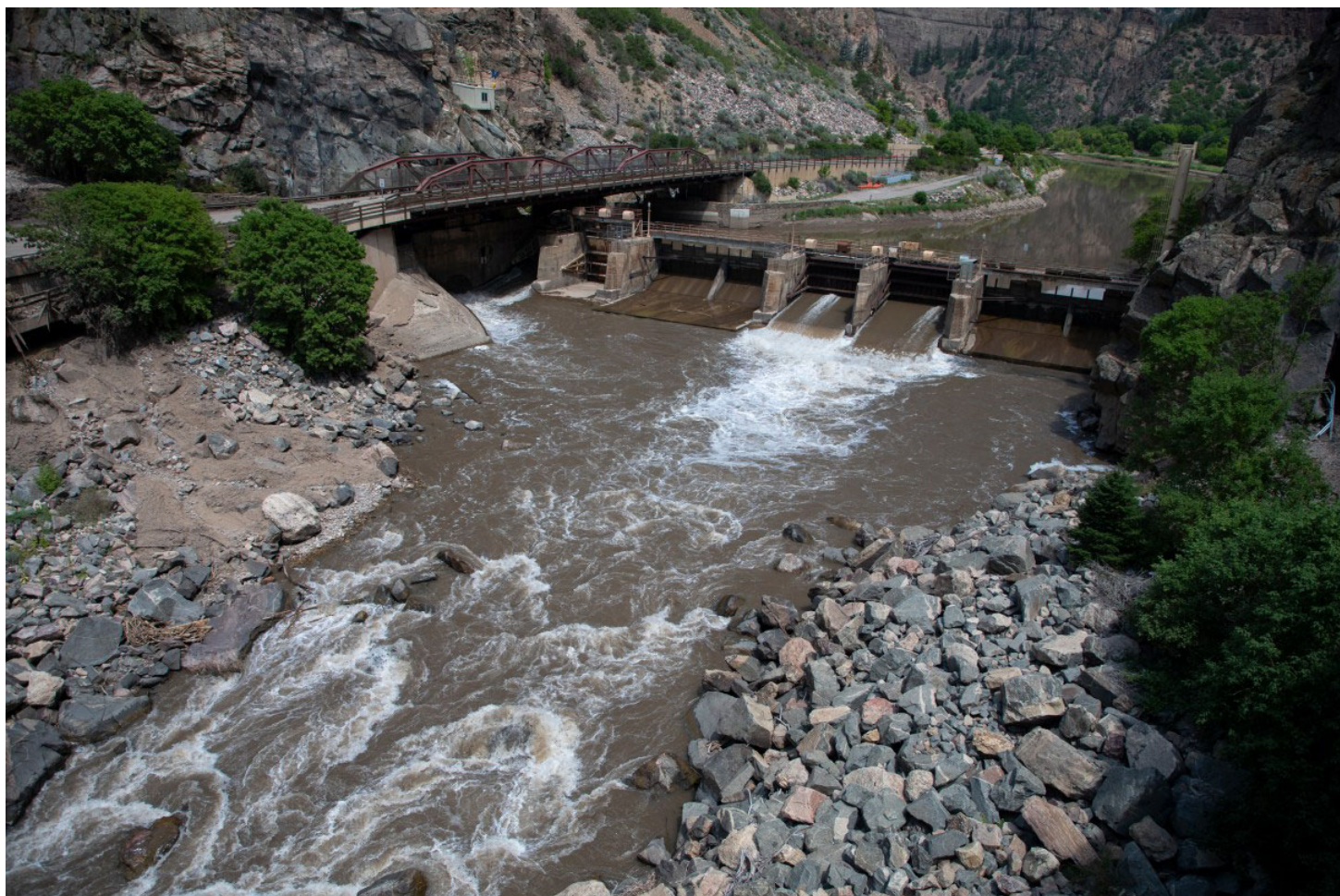
Shoshone Dam, here on August 13, 2021, near Glenwood Springs, is generating electricity through its turbines on the Colorado River. The dam and power plant near the Hanging Lake parking area was constructed in the early 1900s. (Hugh Carey, The Colorado Sun)
