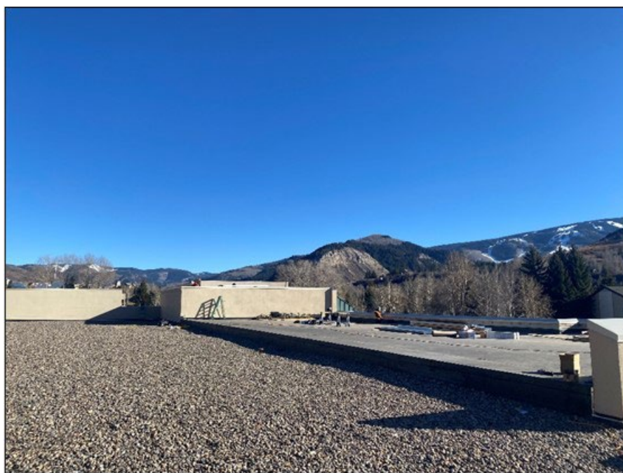
ADWF roof installation
