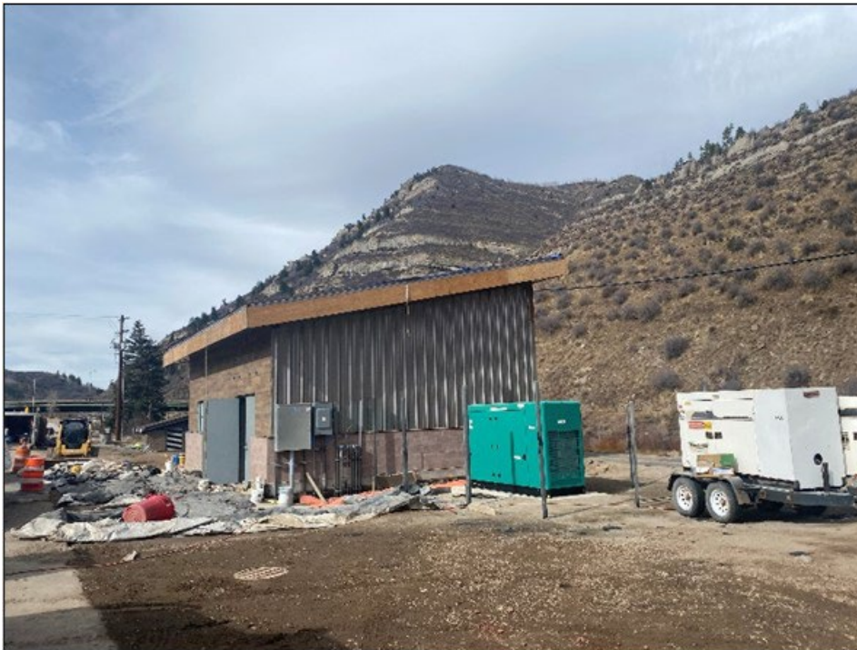
Lift station siding and generator installation
