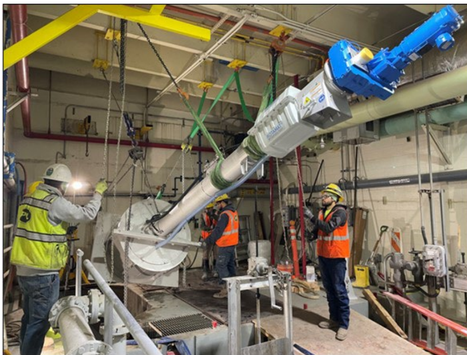
Installation of new barscreen
