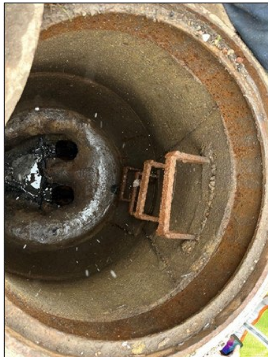
Siphon manhole with both barrels visible
