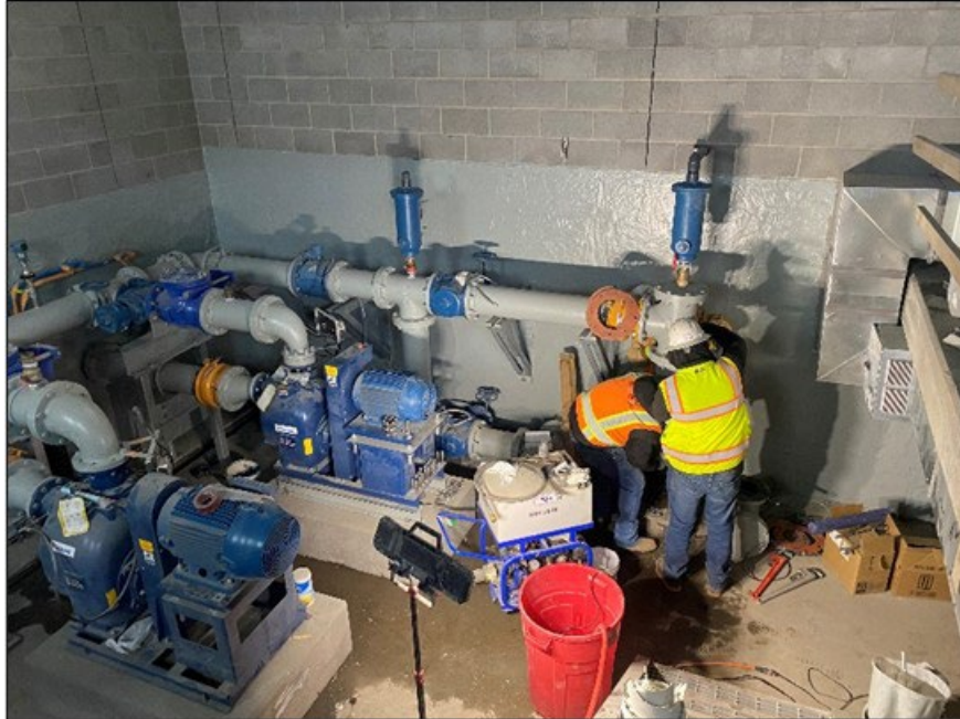
Process piping tie-in after a successful pressure test
