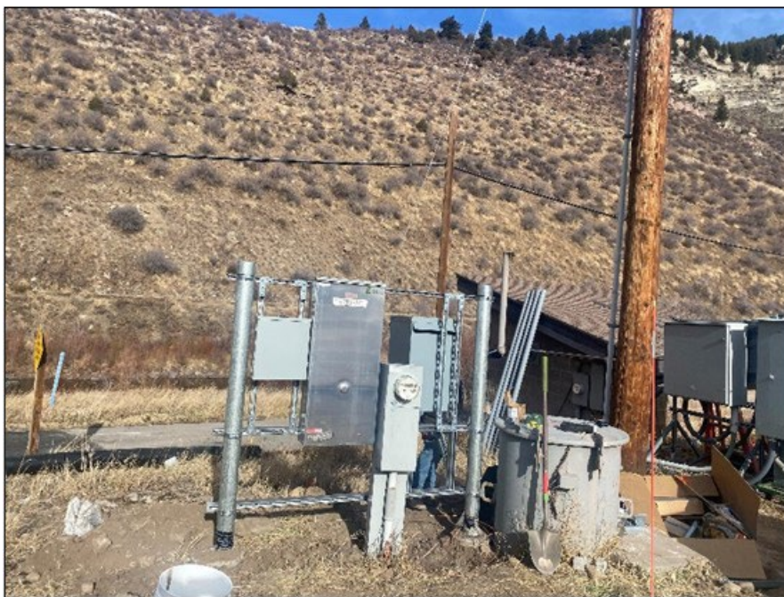
Preparation for the upcoming electrical service tie-in
