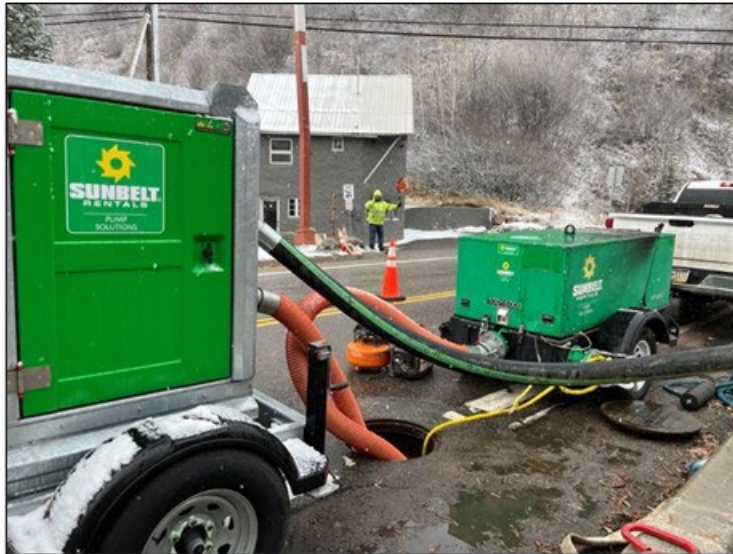
Bypass pump setup on Highway 24 in Minturn
