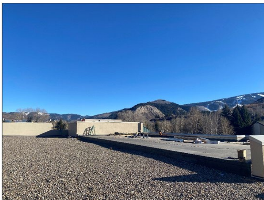
ADWF roof installation
