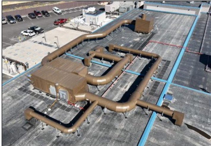
Final coating of HVAC and ductwork
