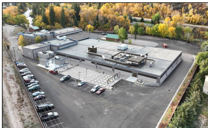
Completed site photo (view looking southeast)
