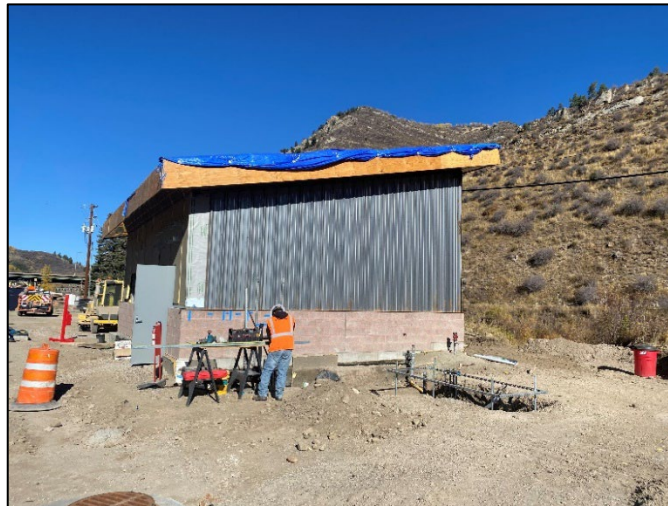
Siding installation at the lift station
