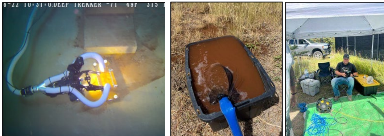
Comprehensive water tank inspection and cleaning performed using an ROV
