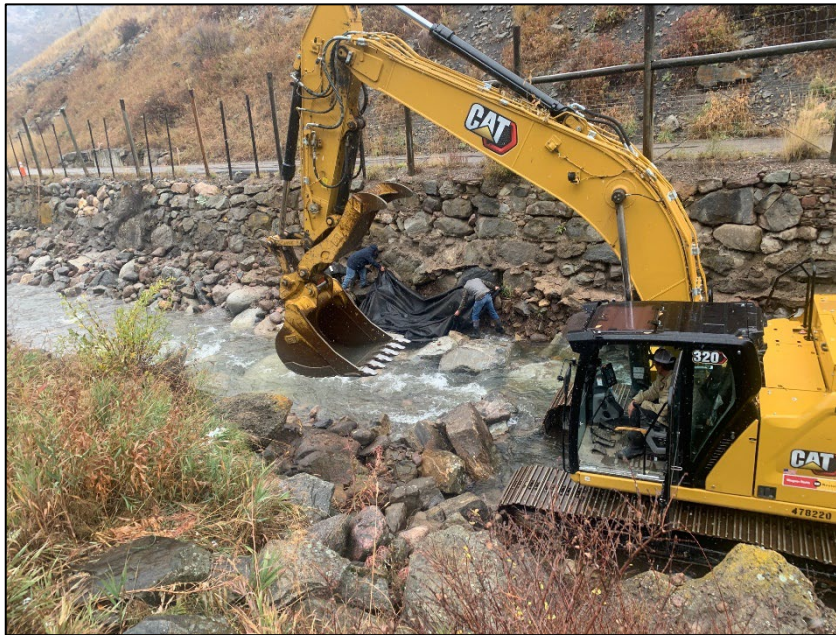
Filter fabric installation on the streambank
