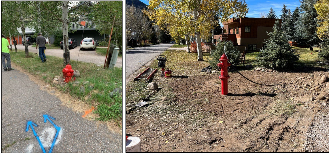
Fire hydrant replacement (before and after)
