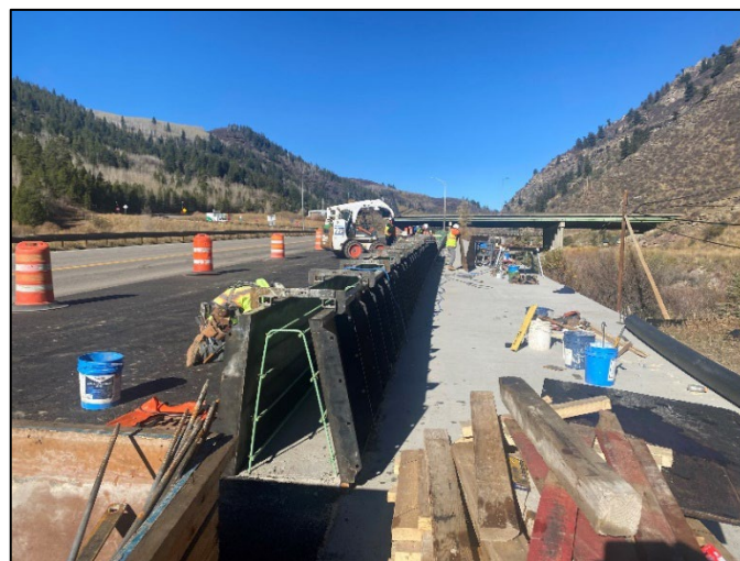
Trail and traffic barrier installation
