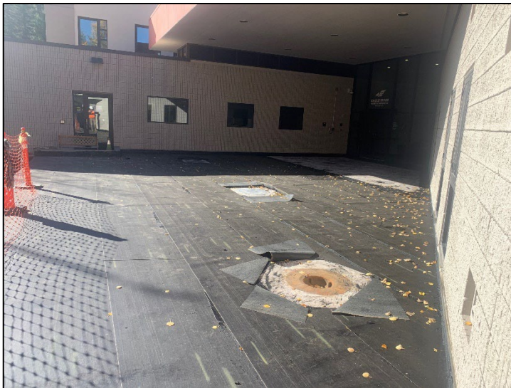
Front plaza waterproofing
