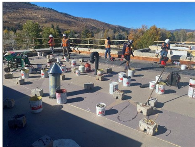
ADWF roof installation progress
