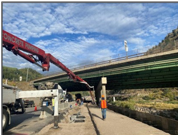
Concrete placement for Eagle County's new bike trail
