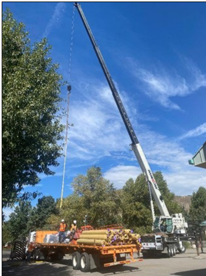
Roof material delivery
