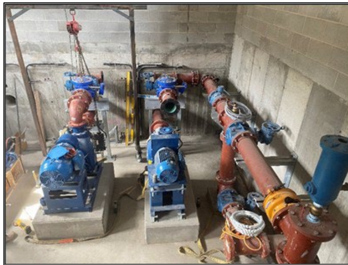
Process piping installation in the new lift station
