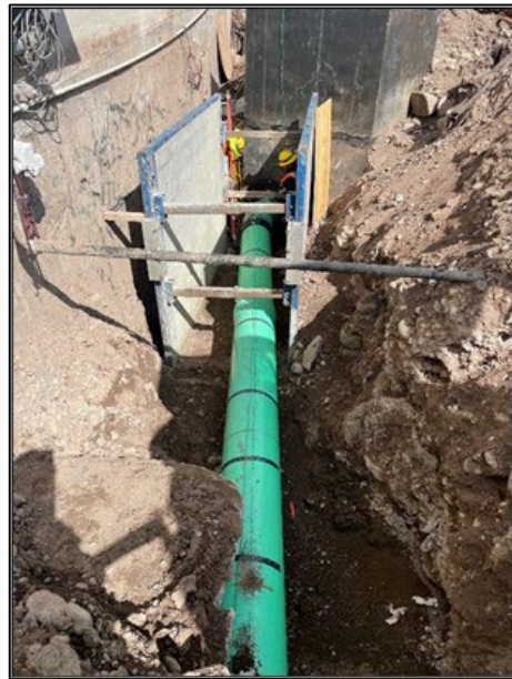
New bypass sewer line
