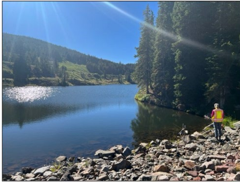
State dam safety engineer inspection of Black Lake No. 2
