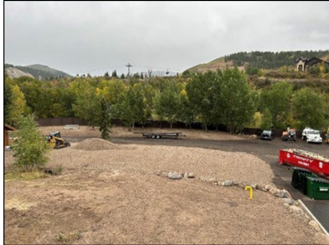
Site work on southwest side of the facility
