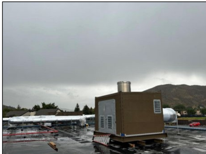
HVAC work on aeration basin roof
