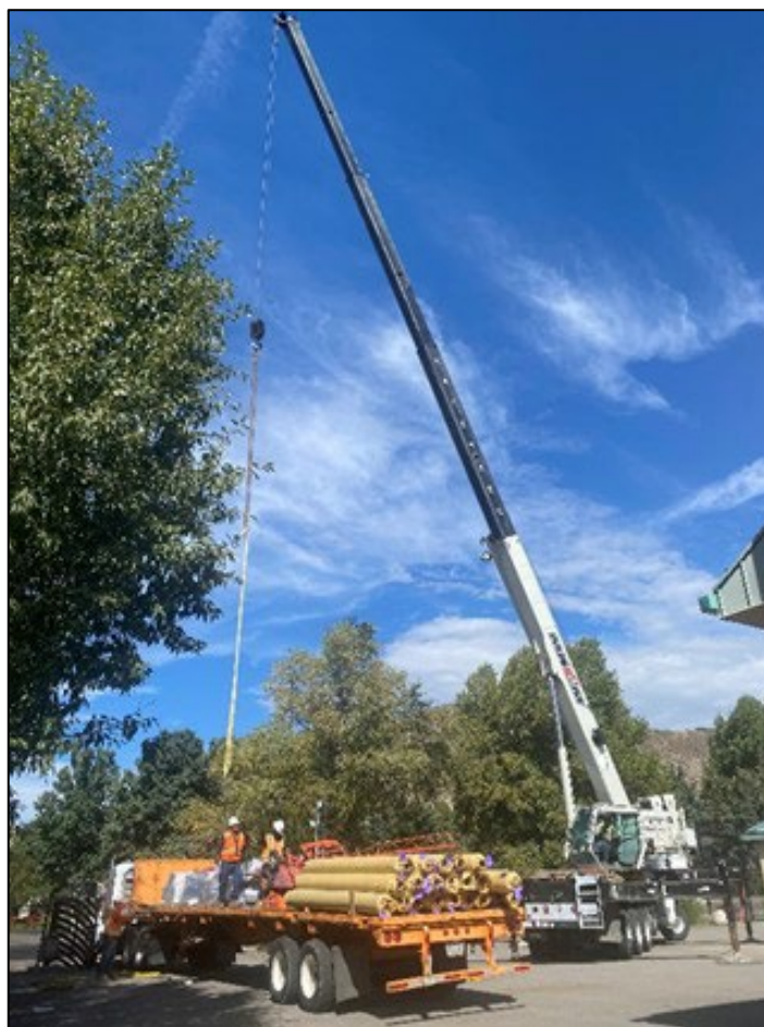
Roof material delivery
