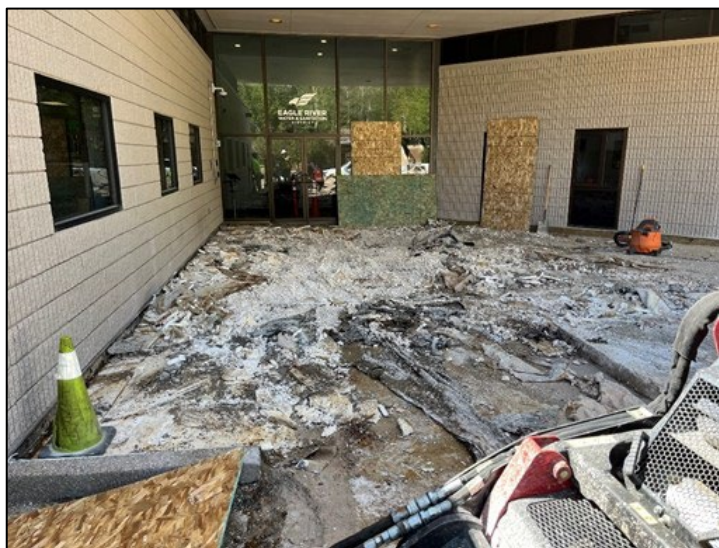
Front plaza demolition
