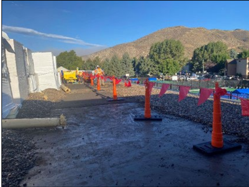
Roofers working on north side of ADWF roof
