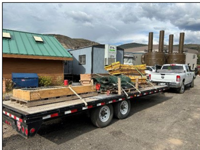
Demobilization of materials from the site
