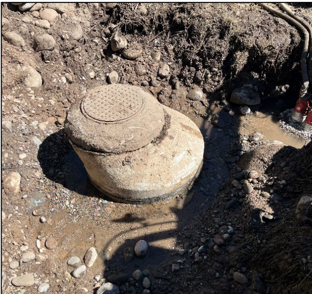
Sewer manhole raising project (near the Edwards Wastewater Treatment Facility)
