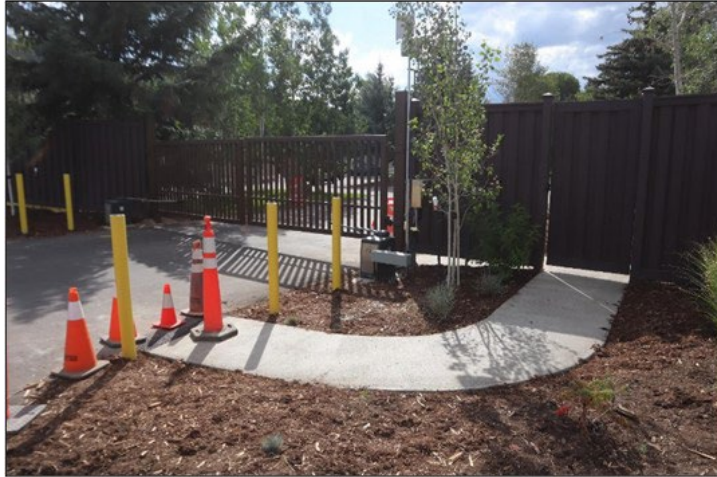
Front entry sidewalk, traffic bollards, and painted fence
