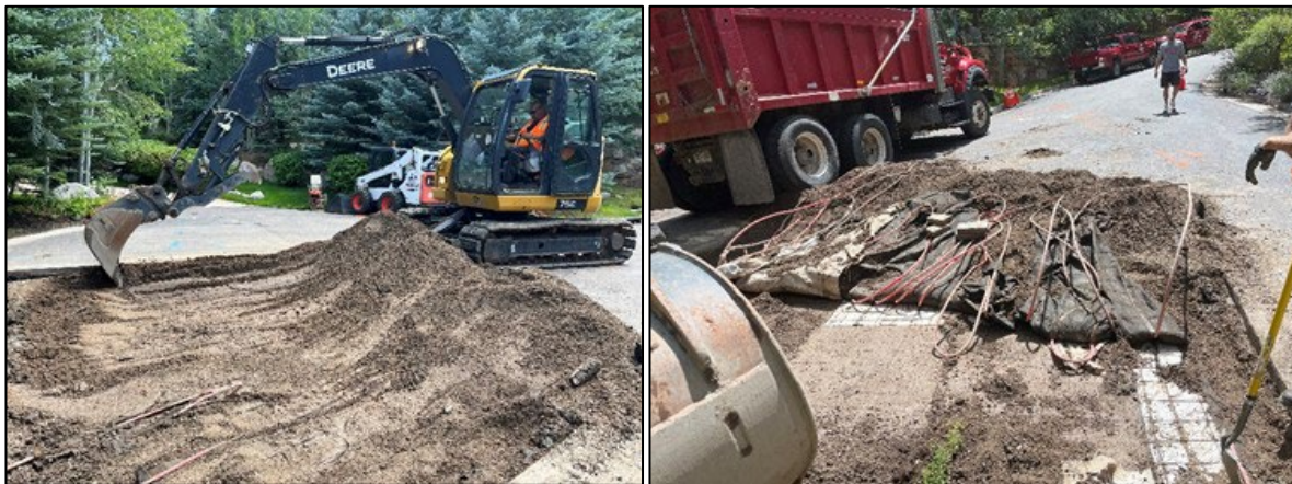
Driveway and heating system removal
