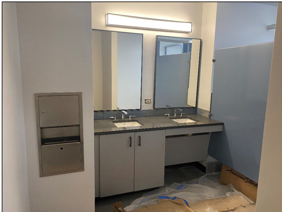
New cabinets, mirrors, and light fixtures in bathroom near Customer Service
