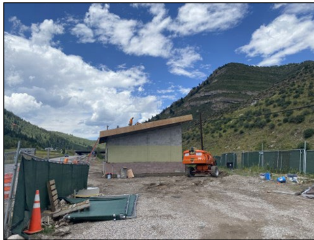
Construction progress at new lift station
