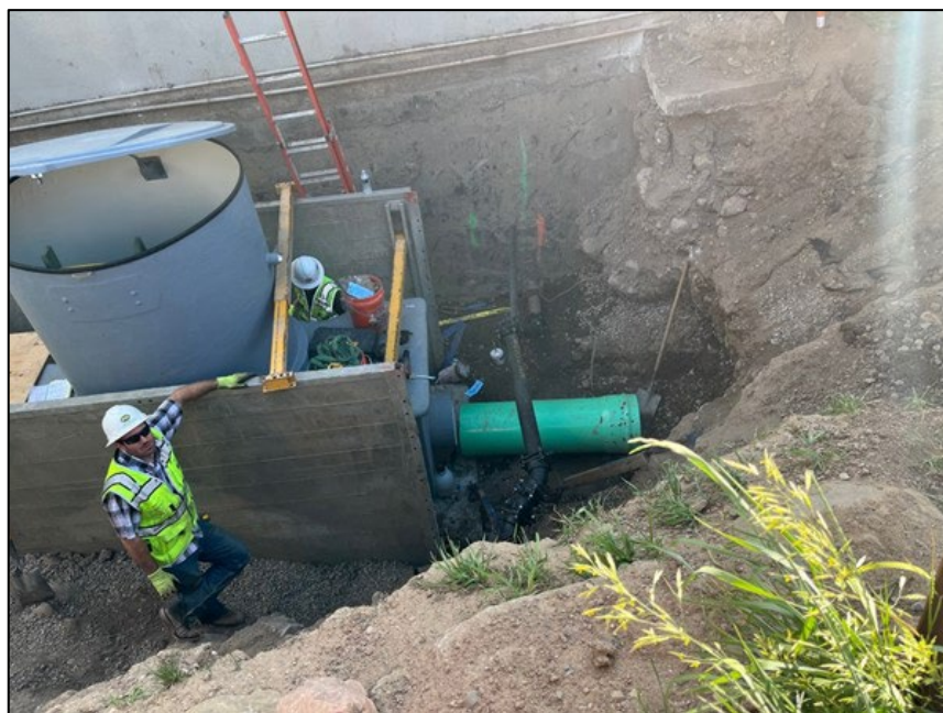
Parshall Flume, Water Service Line, and Sewer Bypass Construction
