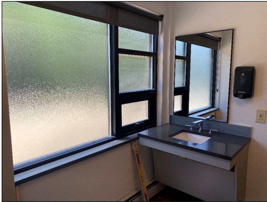
Construction Progress in the Upstairs Women's' Restroom
