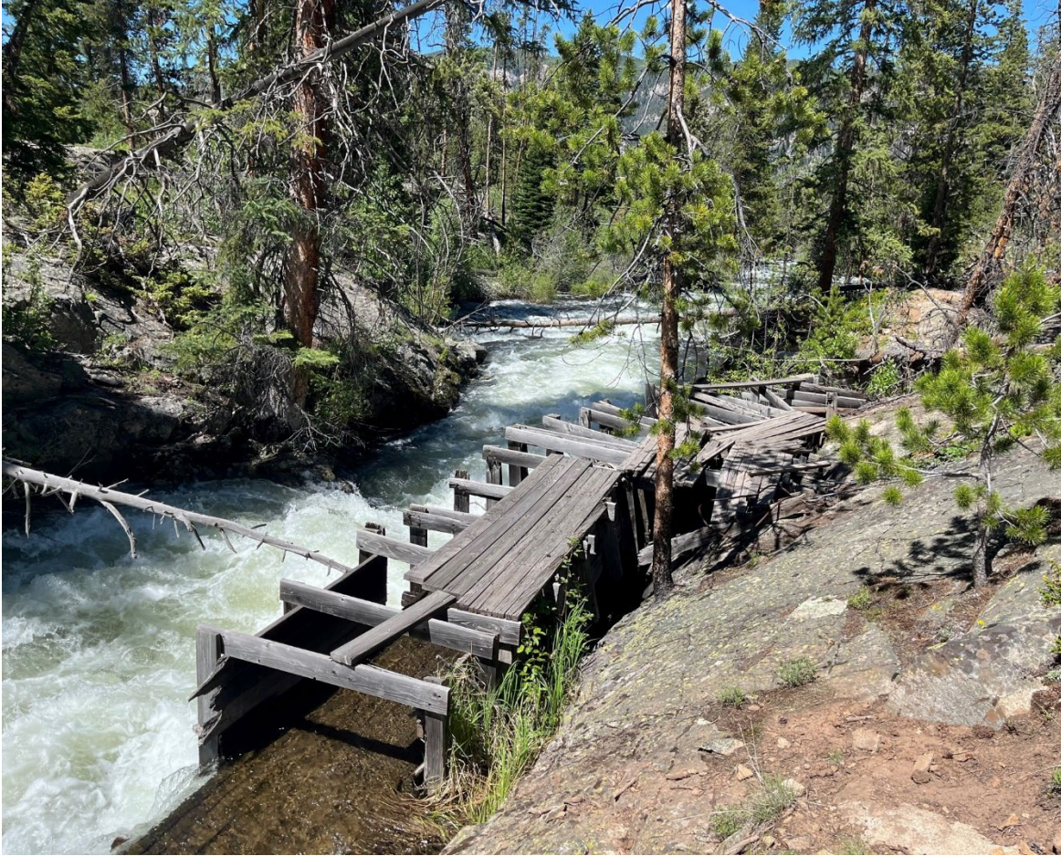
Bolts Ditch Headgate Diversion Structure
