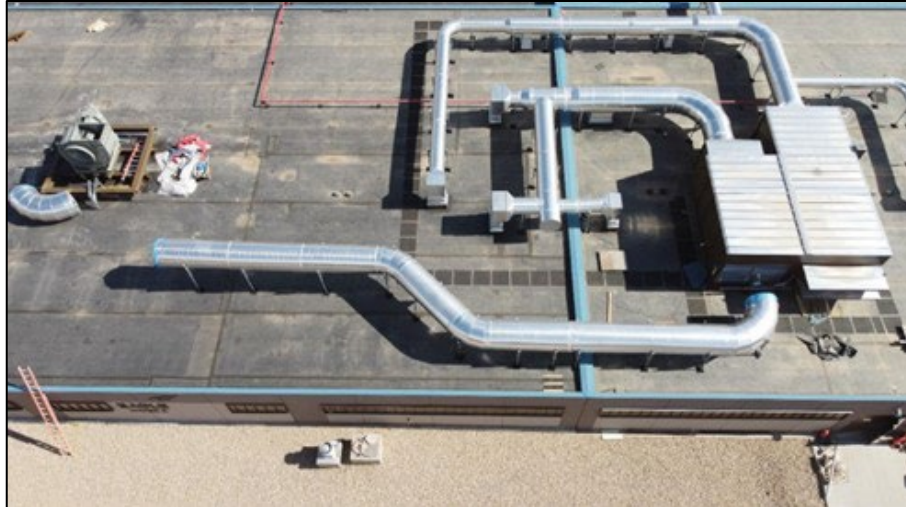
Ductwork Installation on Aeration Basin Building Roof
