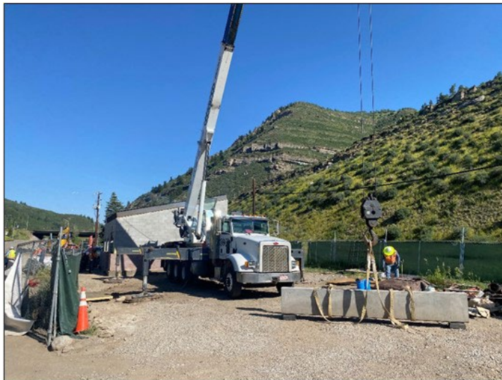
Installation of Lift Station Precast Concrete Structural Beam
