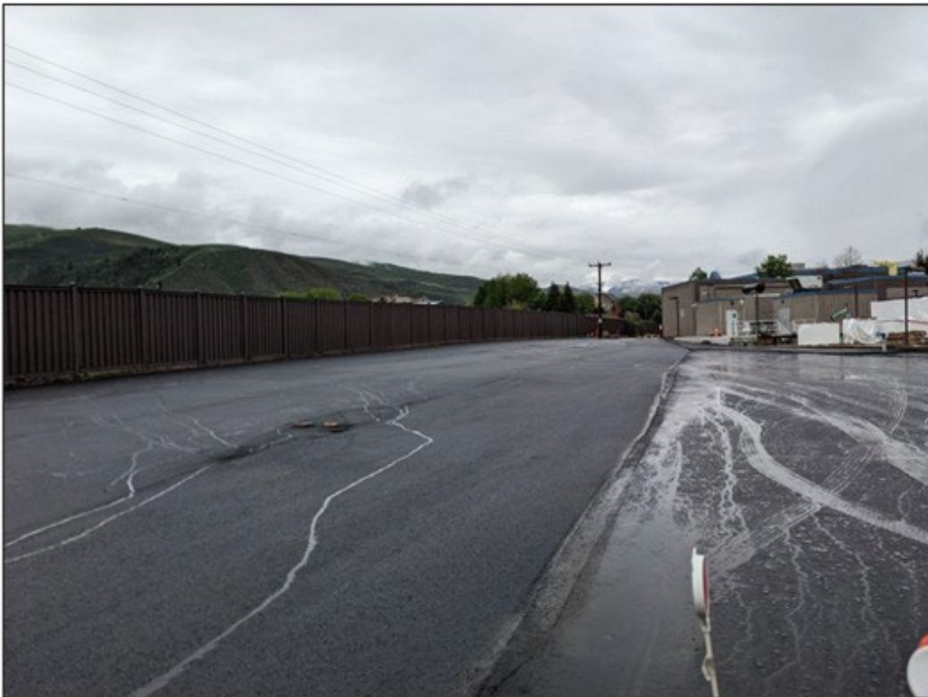
Asphalt Paving – North Side of Site
