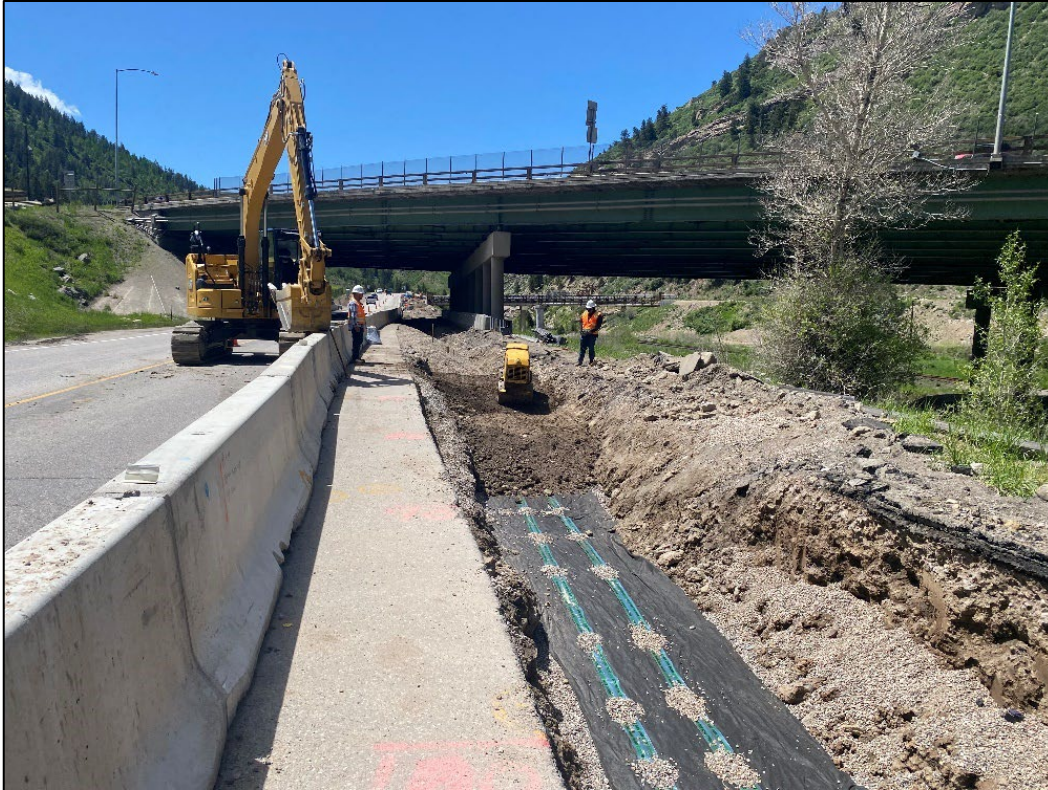
Force Main Installation and Backfill (Southeast of the I-70 Bridge)
