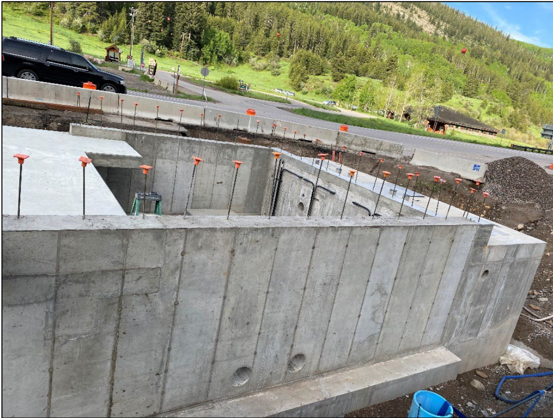
Below-grade Concrete at the New Lift Station
