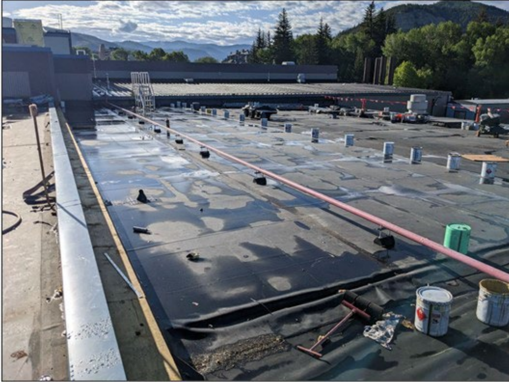
Roof Replacement – Existing Secondary Clarifier Building
