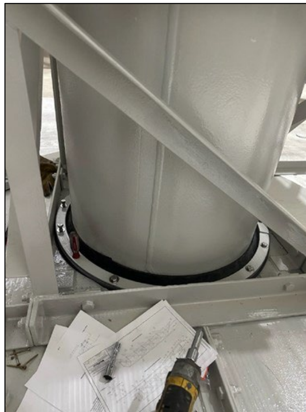
Gasket seal installation on recoated secondary clarifier
