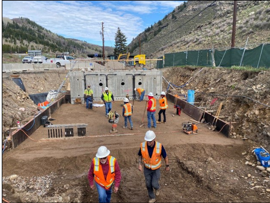
Forming the slab-on-grade for the new lift station dry well
