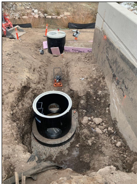
Installation of the sanitary sewer bypass line
