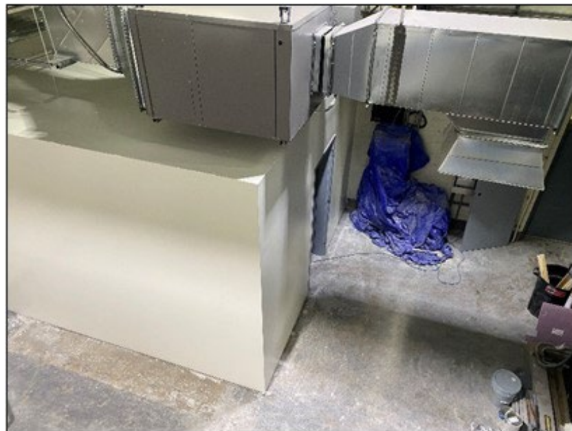
Construction of the new networking and server room
