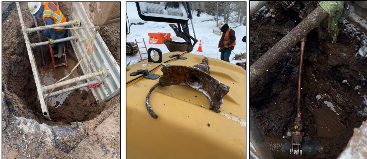
Wildridge water main repair
