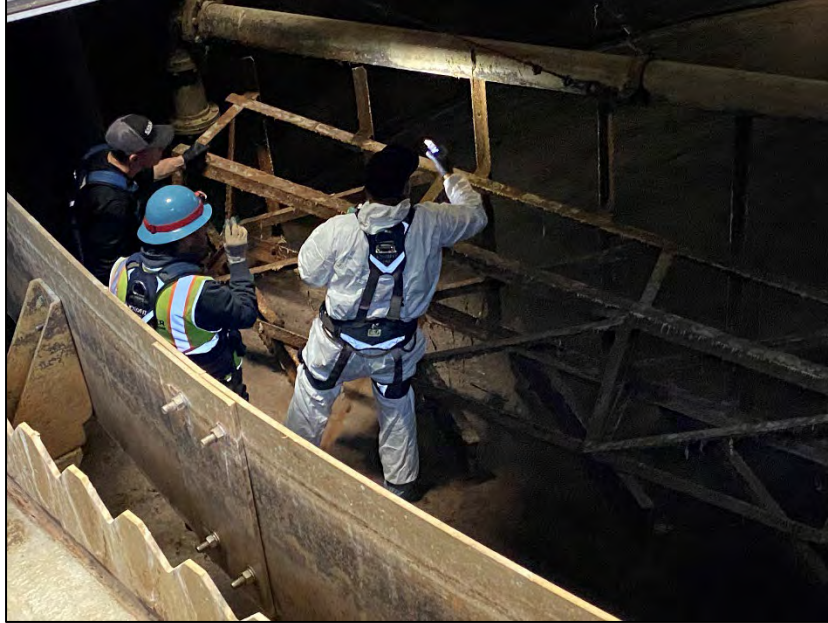
Gravity thickener inspection at the Edwards Wastewater Treatment Facility
