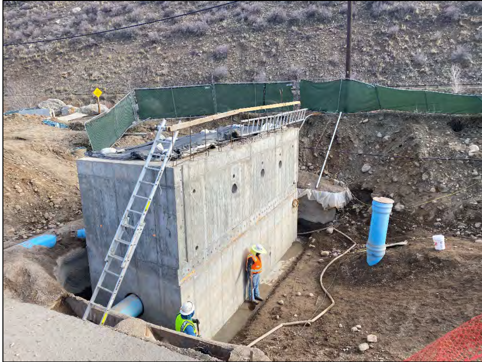
Wet well inspection during hydrostatic leak test
