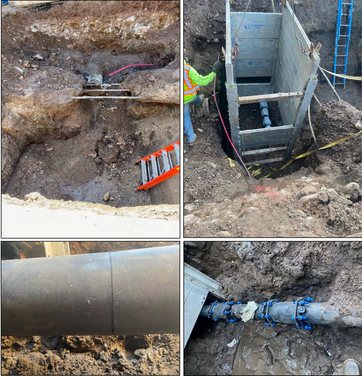
S. Frontage Rd. water main repair
