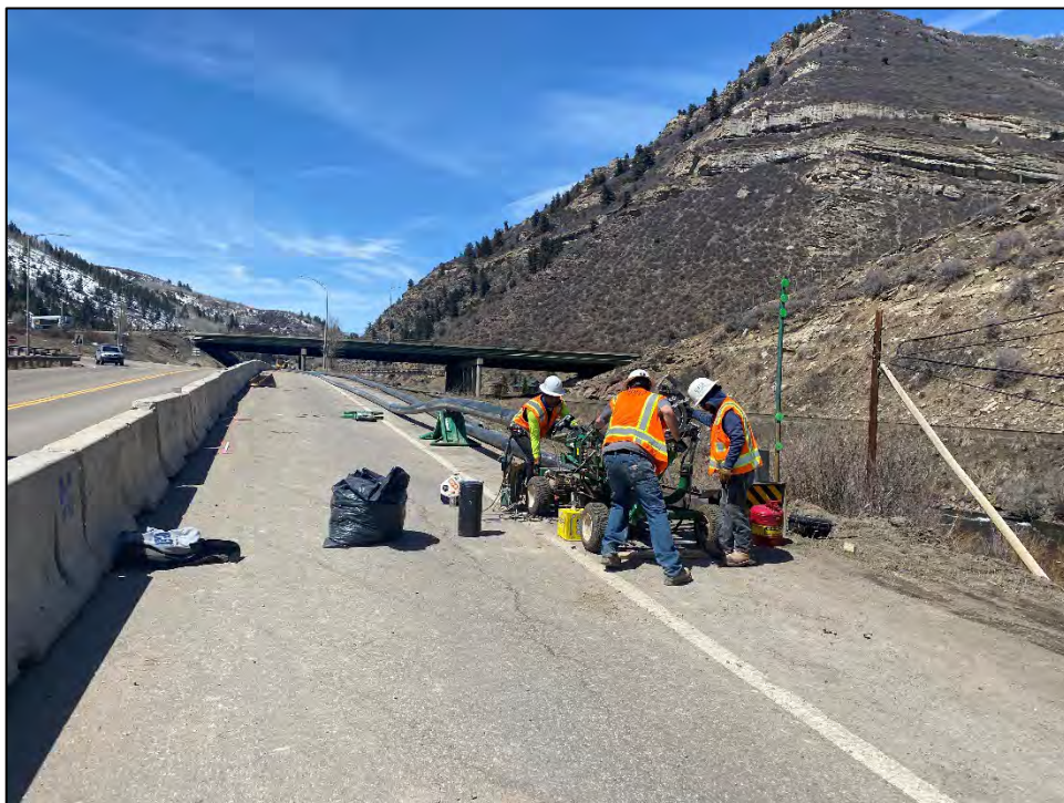
Contractors fusing the HDPE pipe for the new force main
