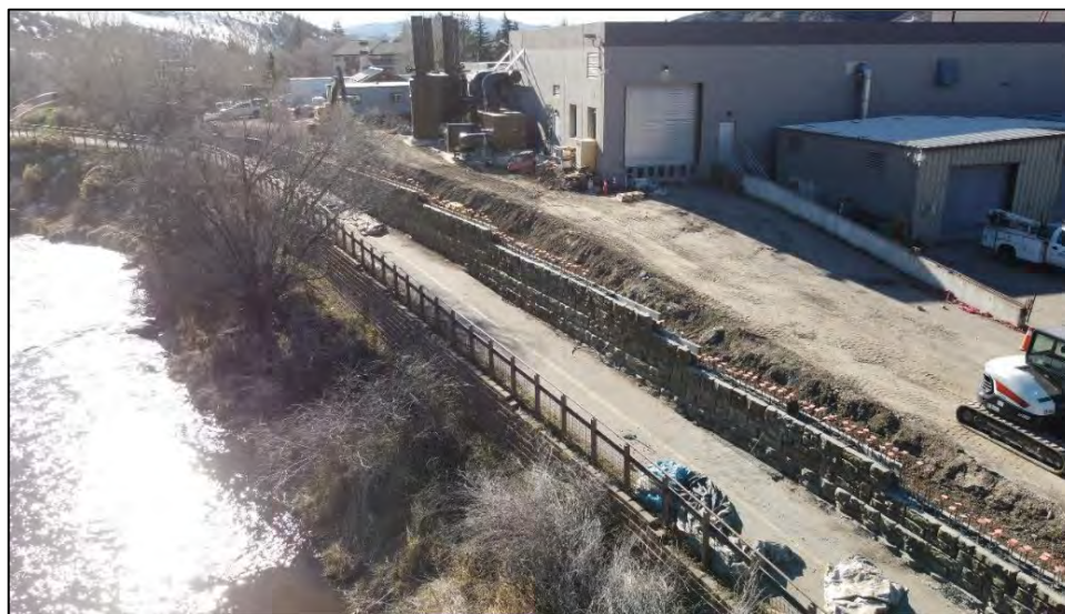
Construction of the retaining wall along the southern property line
