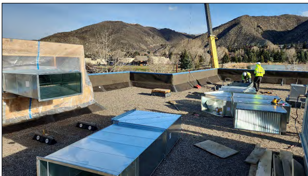
Rooftop duct work/HVAC equipment installation
