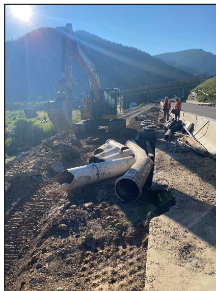
Demolition of the old gravity sewer line (prior to trail construction)
