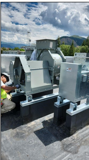
Exhaust fan installation for new lab equipment.
