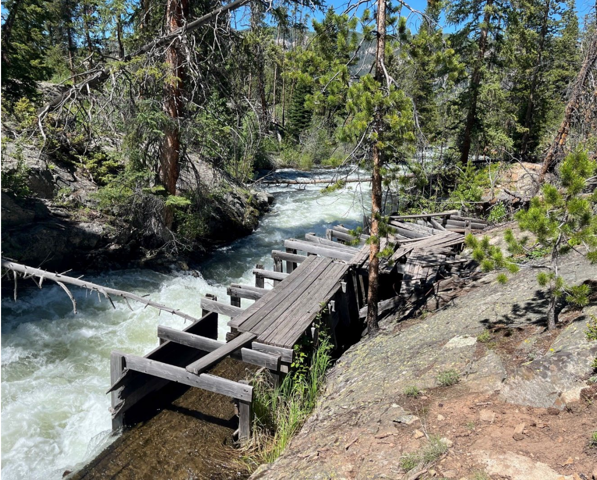
Bolts Ditch Headgate Diversion Structure
