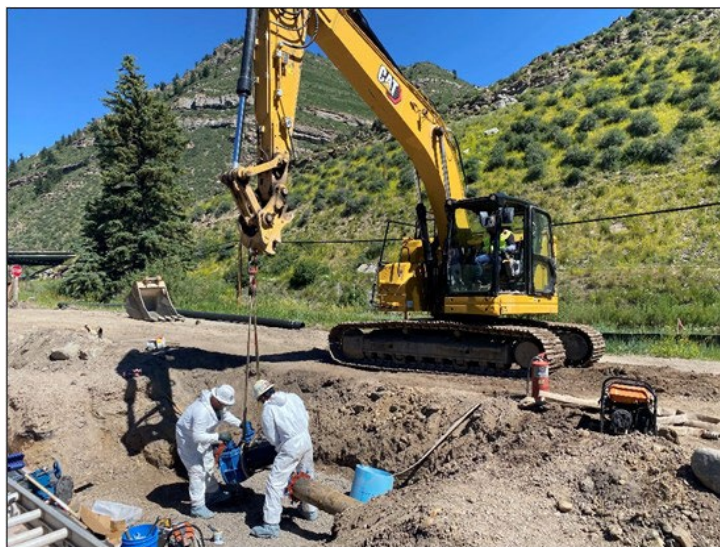
Force Main Pipe Installation
