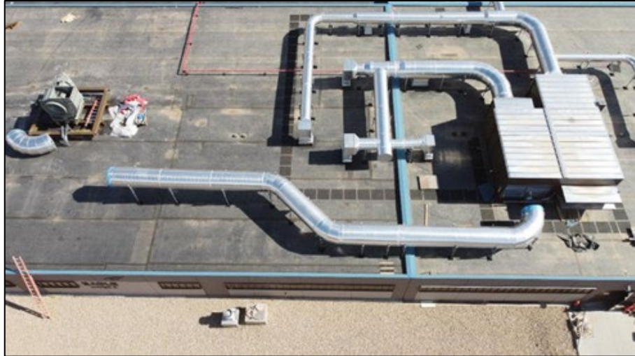
Ductwork Installation on Aeration Basin Building Roof
