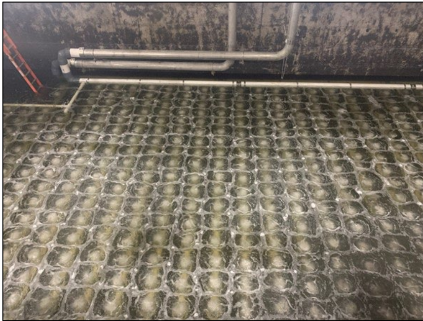
Commissioning of New Aeration Basin Diffusers
