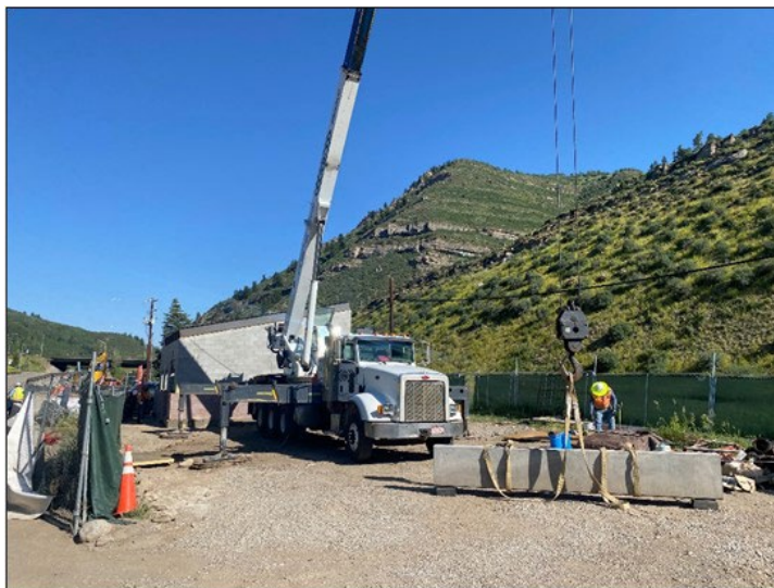
Installation of Lift Station Precast Concrete Structural Beam
