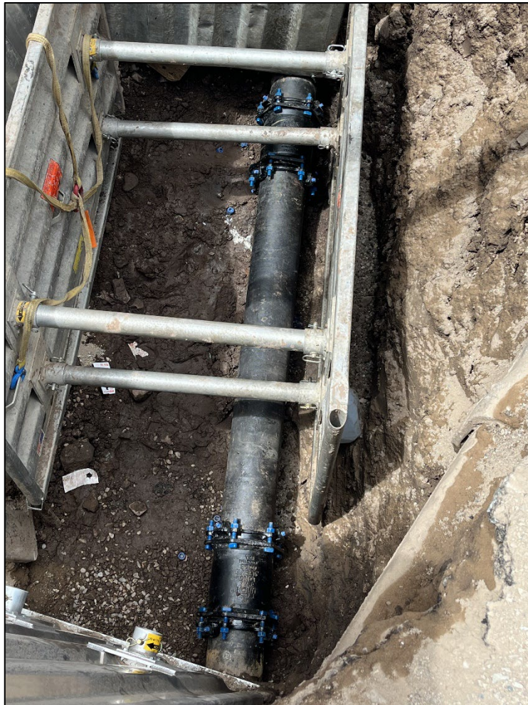
Vail Water Main Repair (Jul. 13-14)
