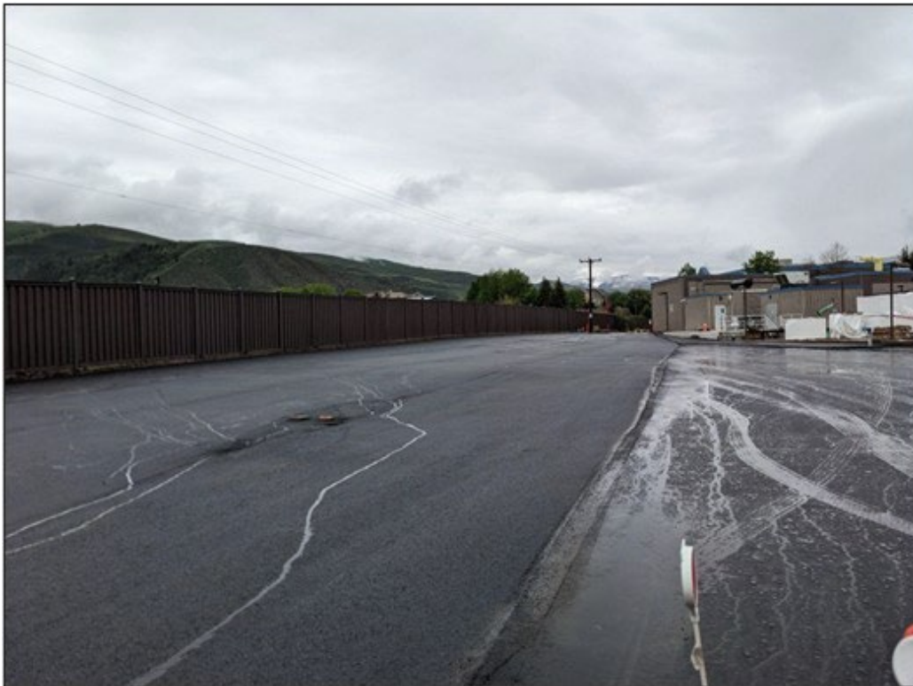
Asphalt Paving – North Side of Site
