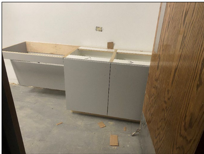
Bathroom Cabinet Installation
