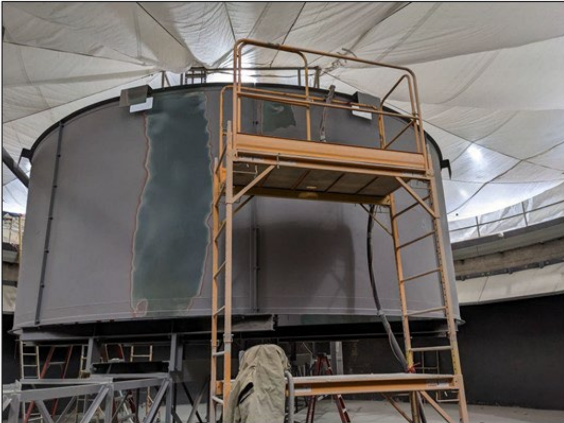
Sandblasting Secondary Clarifier
