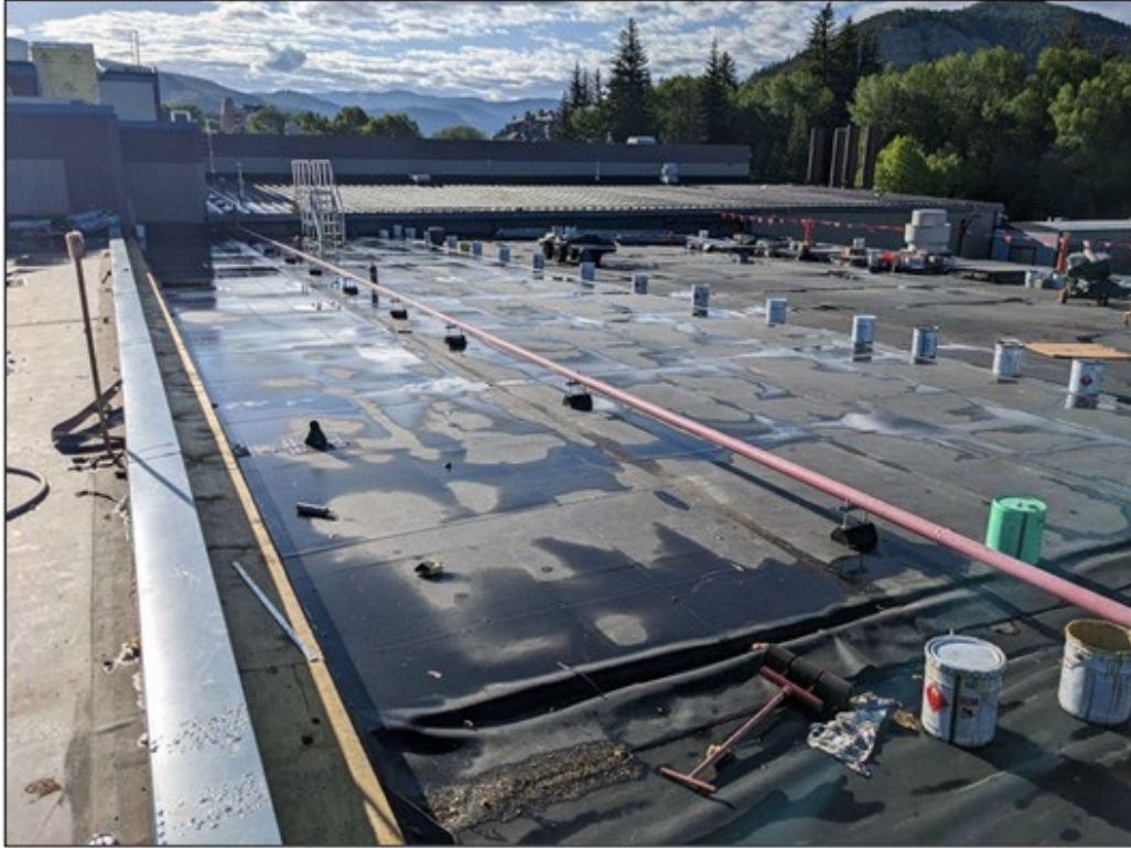
Roof Replacement – Existing Secondary Clarifier Building
