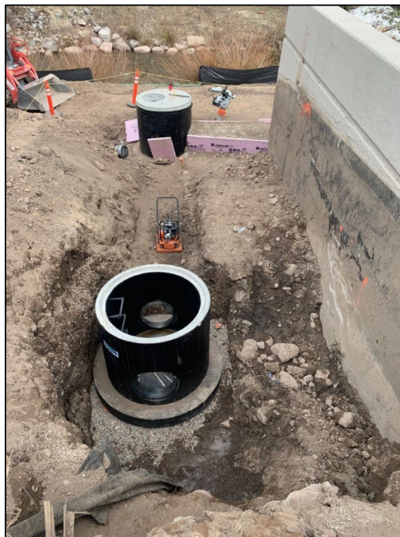
Installation of the sanitary sewer bypass line
