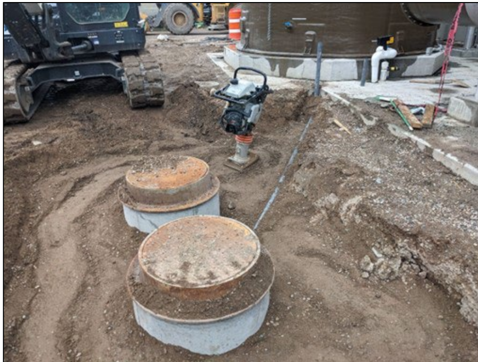
Sand/oil separator backfill, access manholes, and vent system
