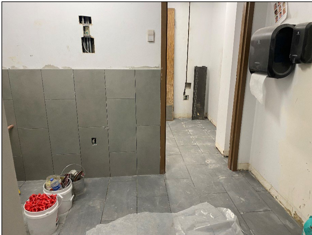
Tile installation in the north first floor restroom
