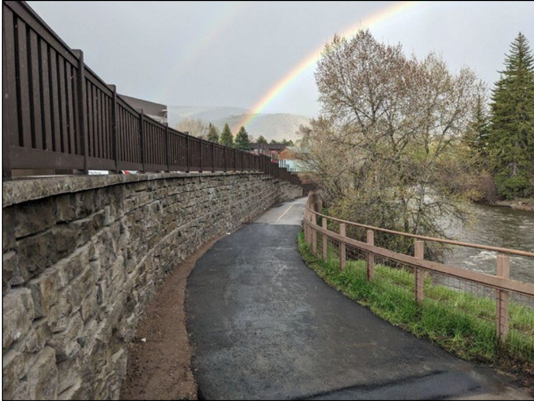
Restored recreation path, retaining wall, and fence
