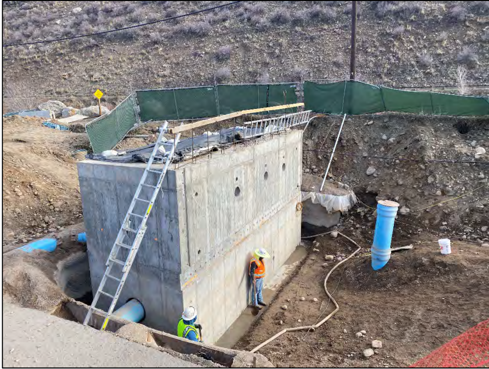
Wet well inspection during hydrostatic leak test
