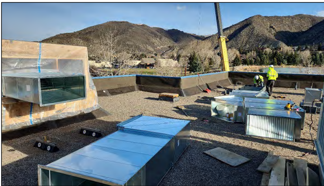
Rooftop duct work/HVAC equipment installation
