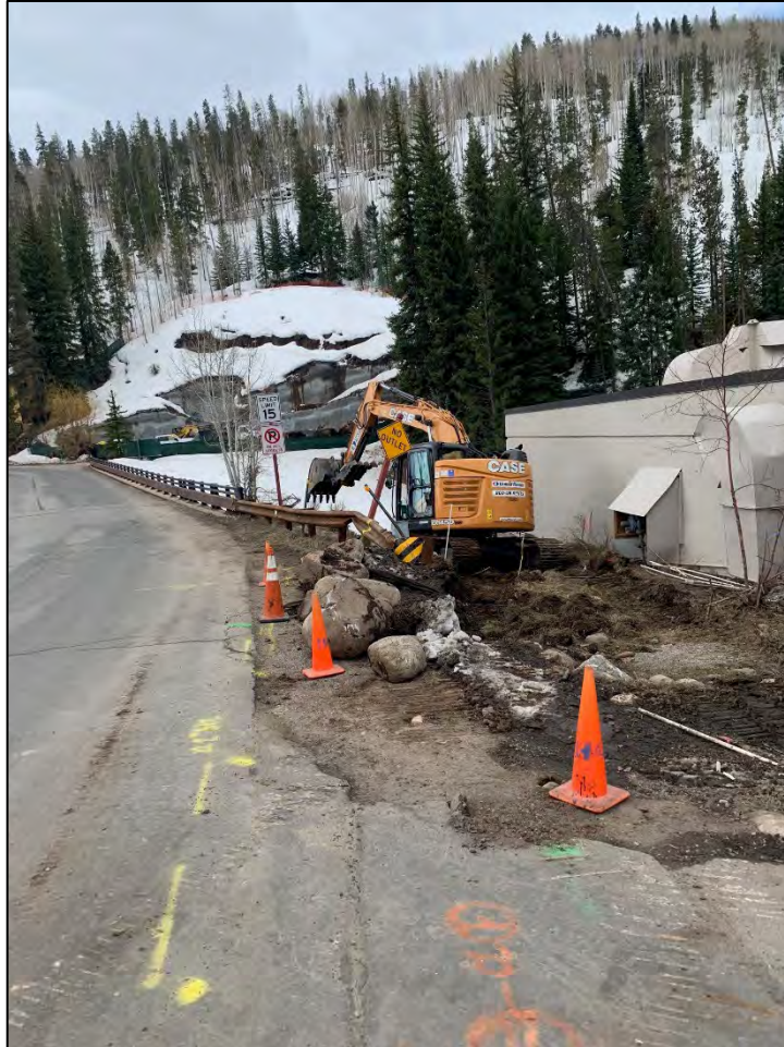
Installation of the sanitary sewer bypass pipe
