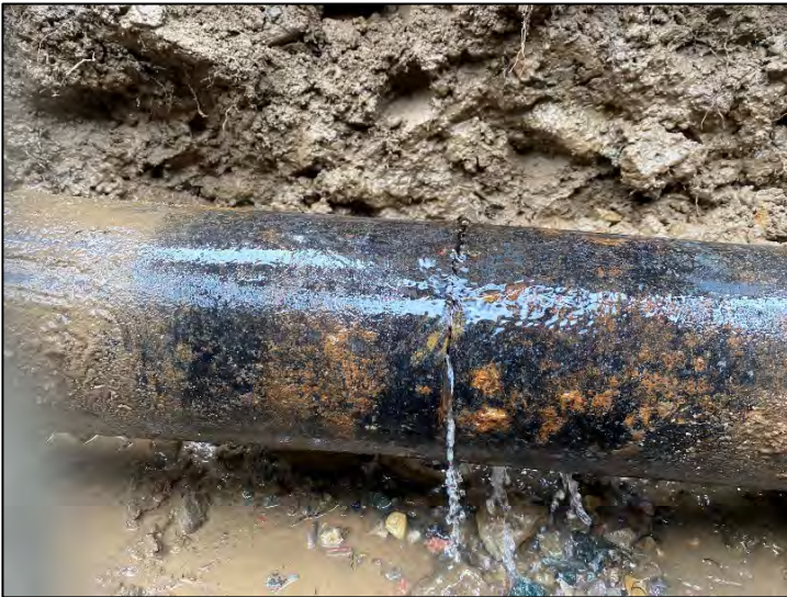
Matterhorn Circle water main repair
