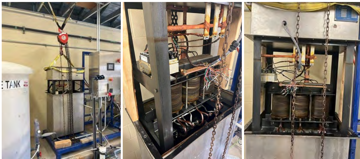
On Site Sodium Hypochlorite Generator (OSHG) repair at Berry Creek Wellhouse
