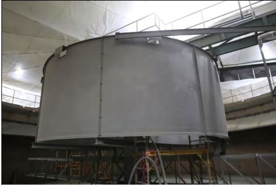
Recoating work in clarifier
