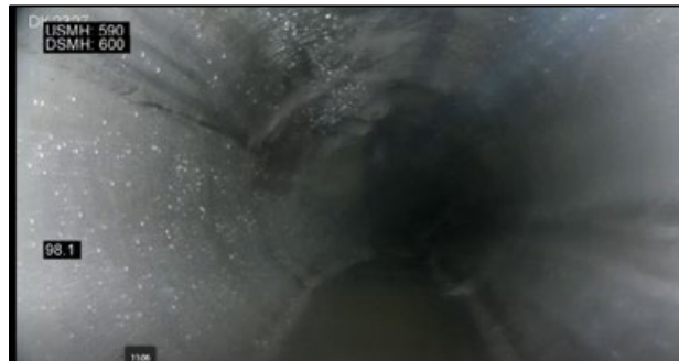
Avon sewer interceptor rehabilitation (damaged pipe before repairs left, rehabilitated pipes with CIPP liners right)
