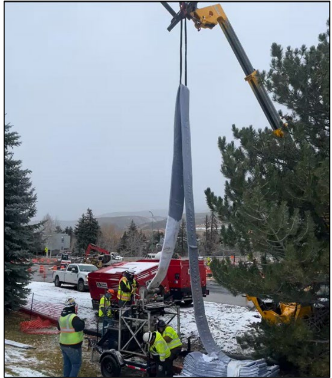
Avon sewer interceptor construction activities (bypass piping left, CIPP liner installation right)
