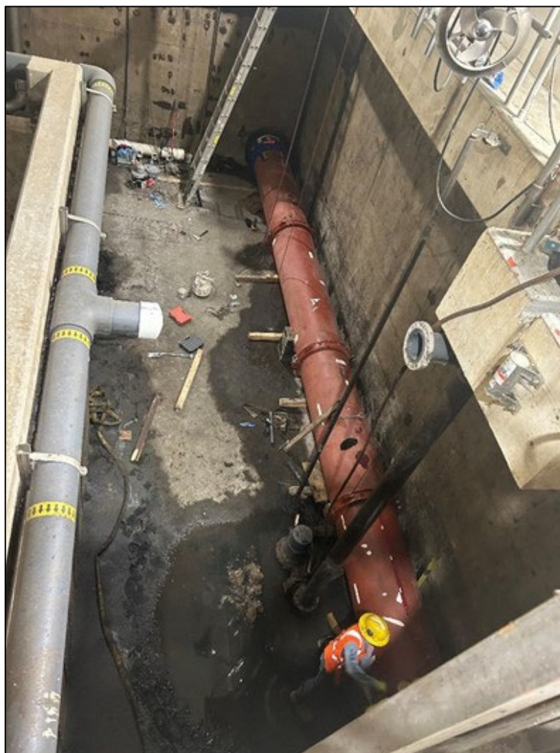
Mixed liquor pipe replacement at VWW (new pipe shown on right side of photo)
