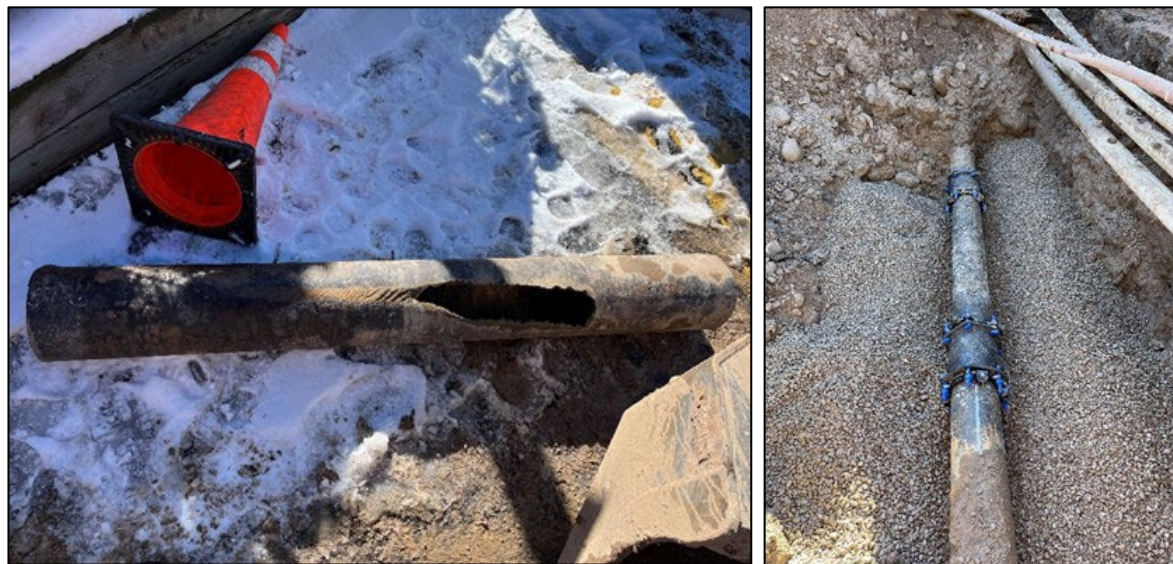
West Beaver Creek Blvd. water main repair (damaged pipe left, completed repair right)
