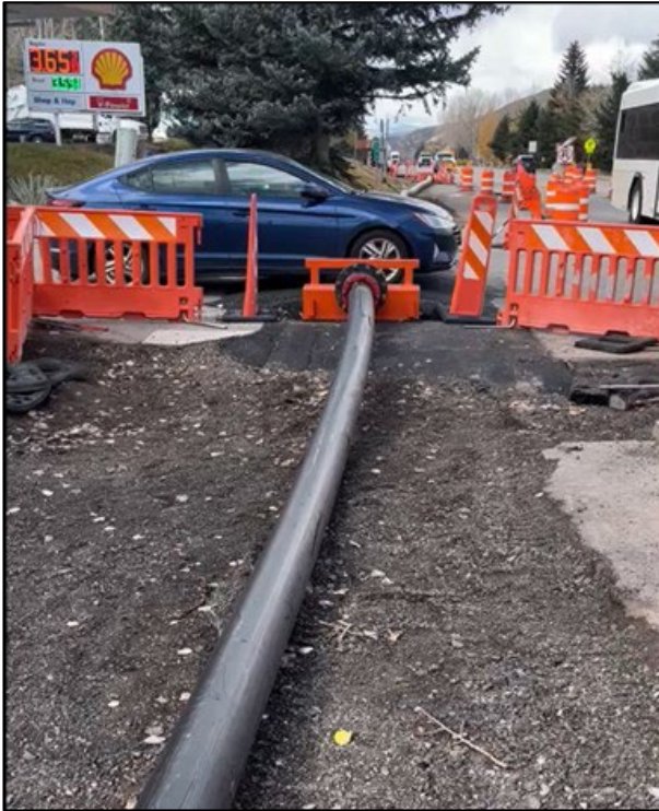
Avon sewer interceptor construction activities (bypass piping left, CIPP liner installation right)
