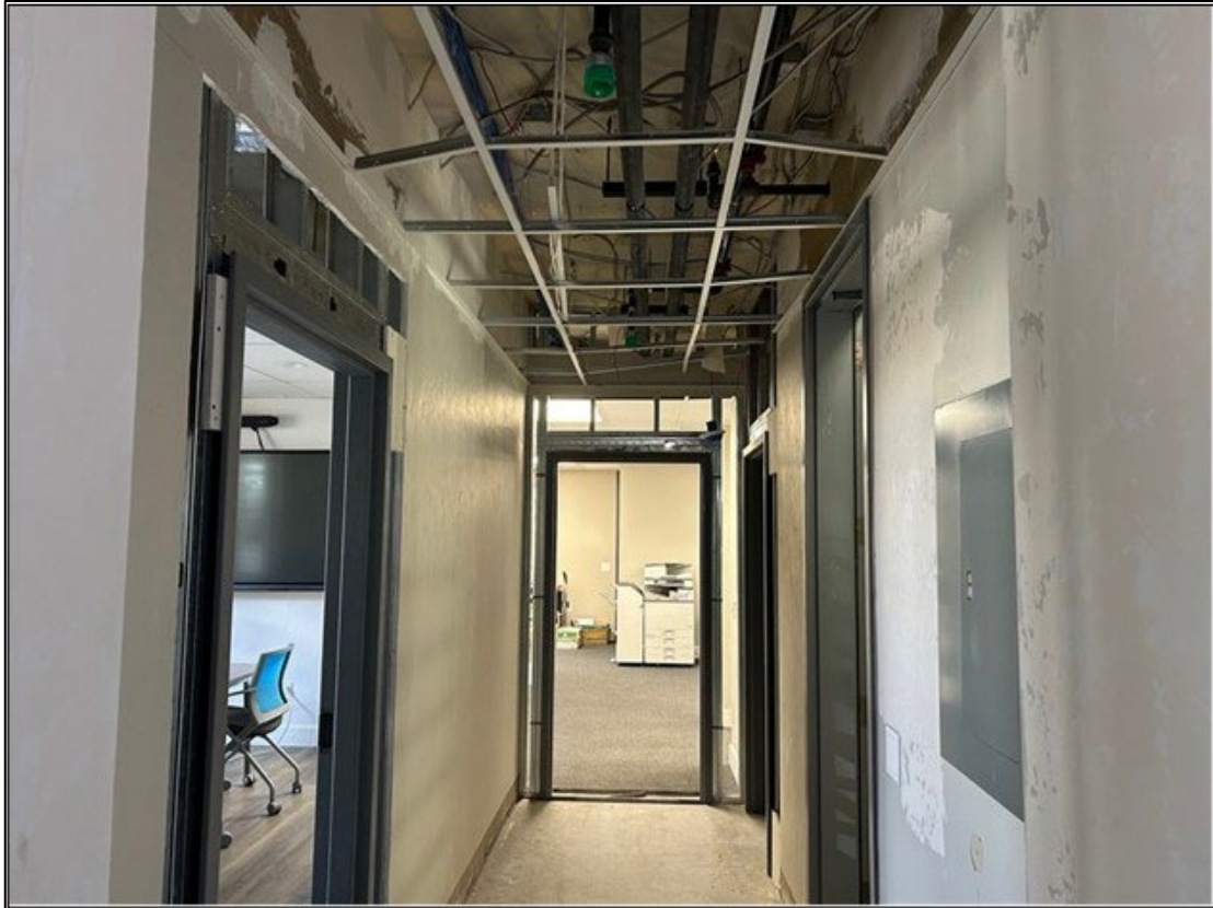
Eagle Vail Office framing and fire sprinkler installation
