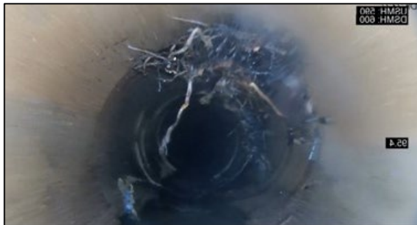
Avon sewer interceptor rehabilitation (damaged pipe before repairs left, rehabilitated pipes with CIPP liners right)
