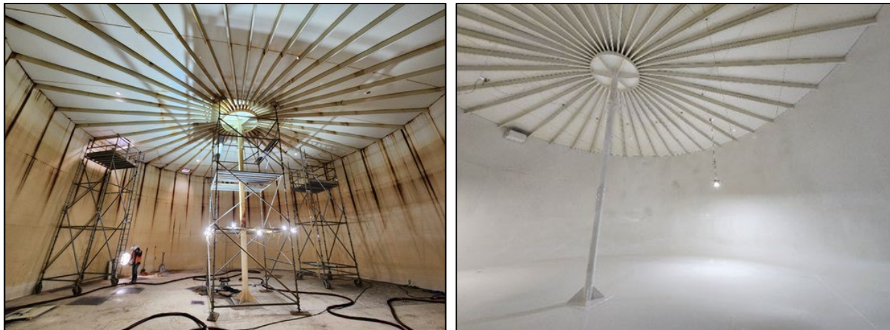
Cordillera West Tank 1 interior re-coating (before left, after right)
