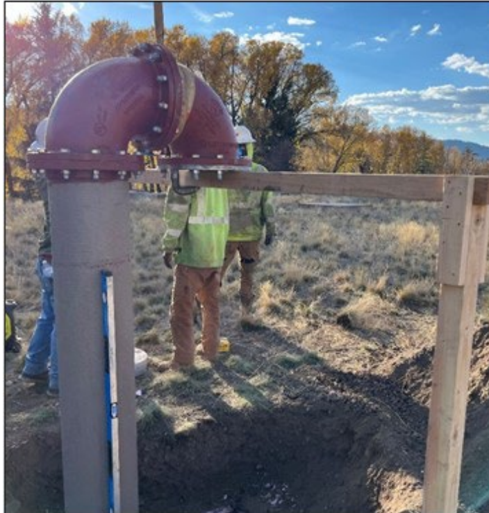
EDWF clearwell vent installation
