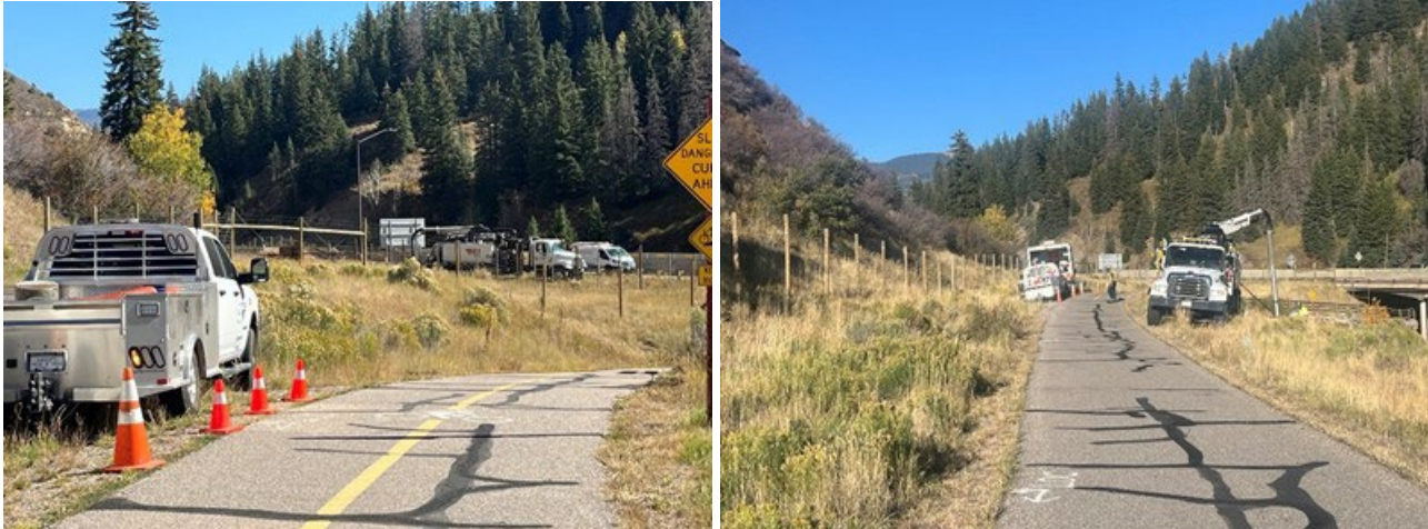
Dowd Junction sewer interceptor cleaning and inspection
