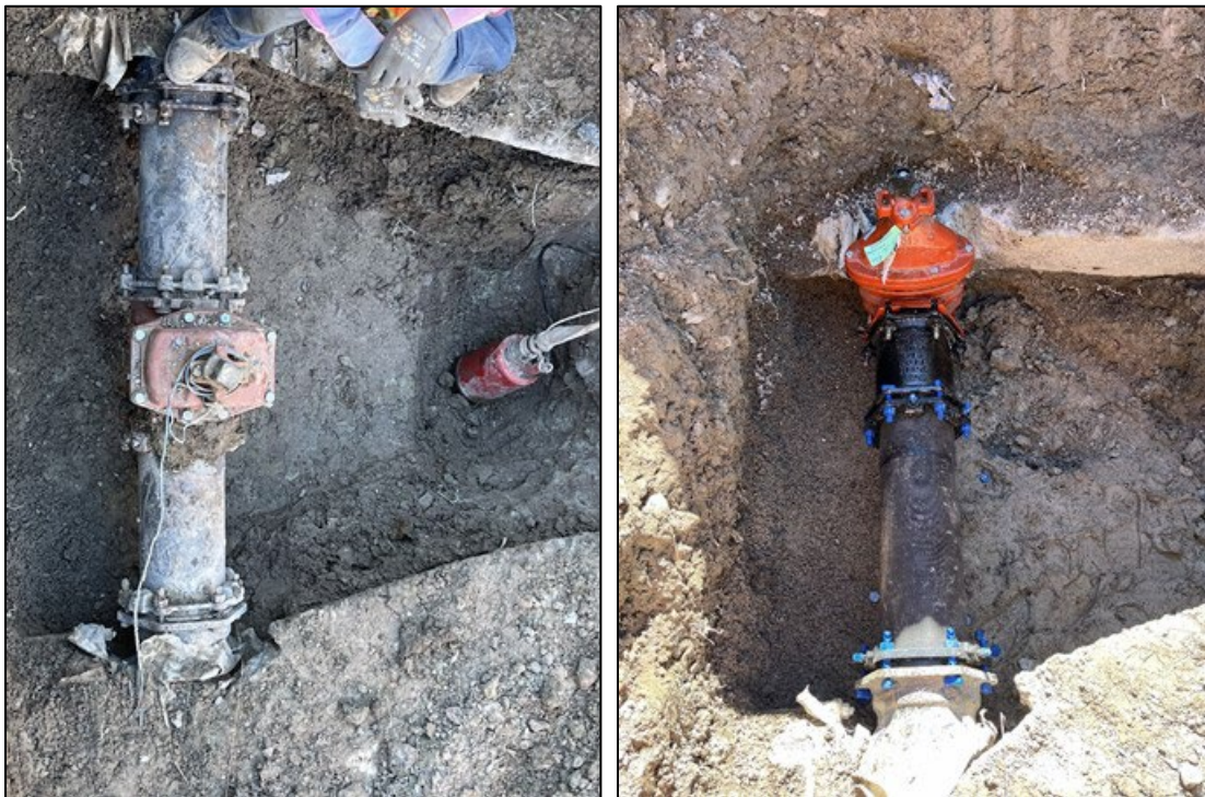
Granada Hill water valve repair (old valve left; new valve right)
