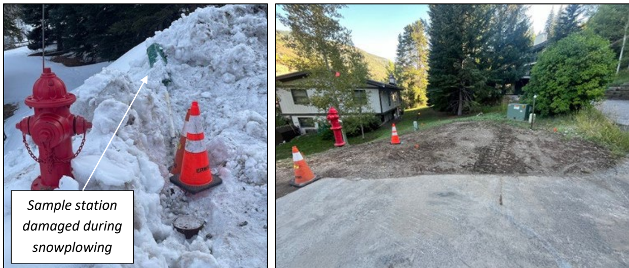
West Vail water sample station abandonment (damaged station left; completed abandonment right)
