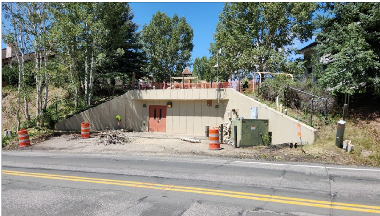
Vegetation removal at Wildridge BPS 2/Tank 1 site
