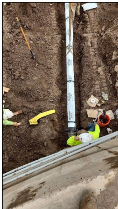
Installation of new overflow pipe at Avon Tank 1
