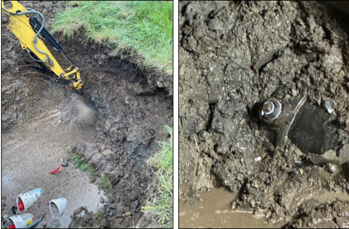
Beaver Creek Golf Course water service repair (excavation and pipe damage left; repair right)
