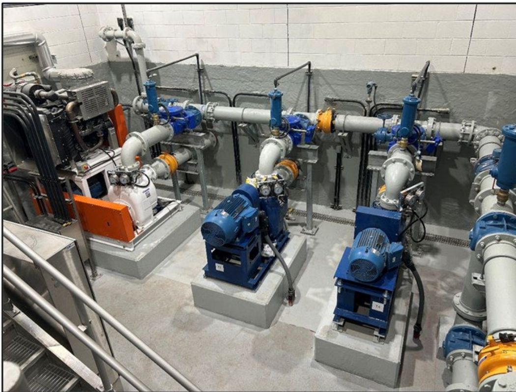
Interior view of completed lift station
