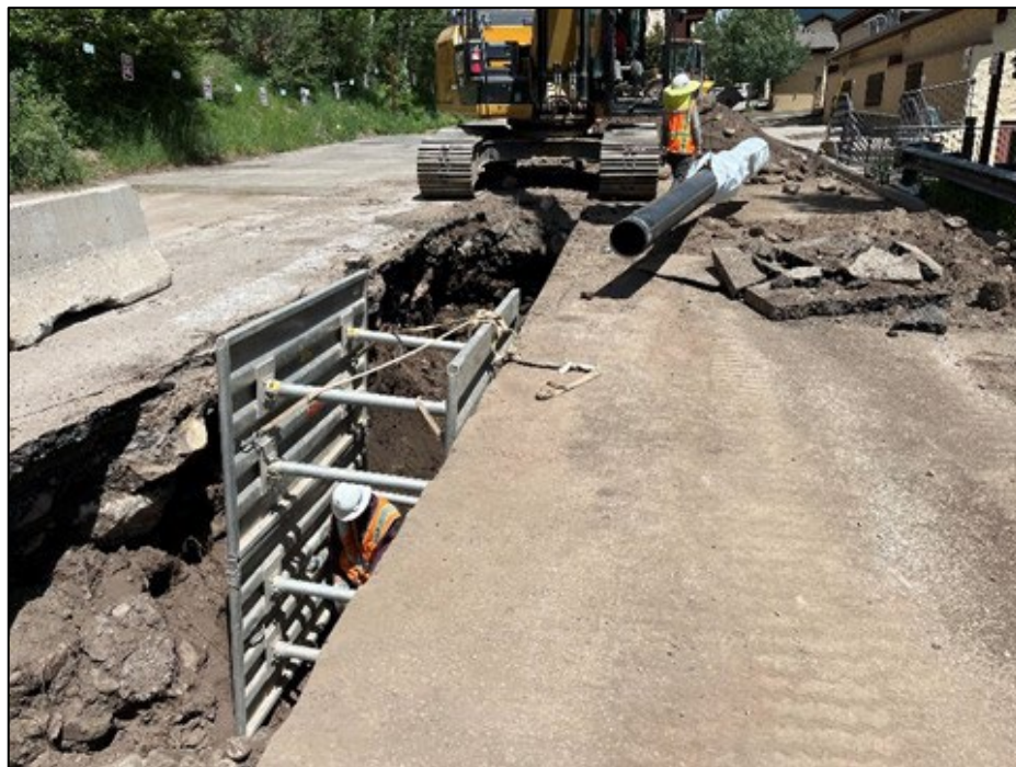
Water main installation along Middle Creek housing access road
