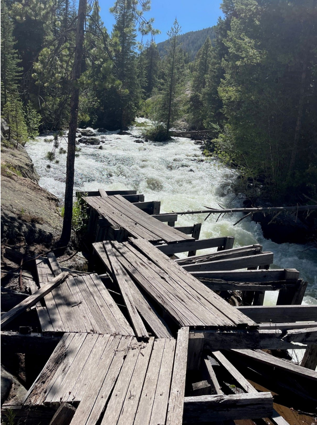
Photograph of Bolts Ditch diversion structure
