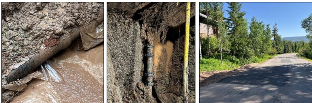
Cordillera water main repair (damaged pipe left, repaired pipe center; completed repair right)
