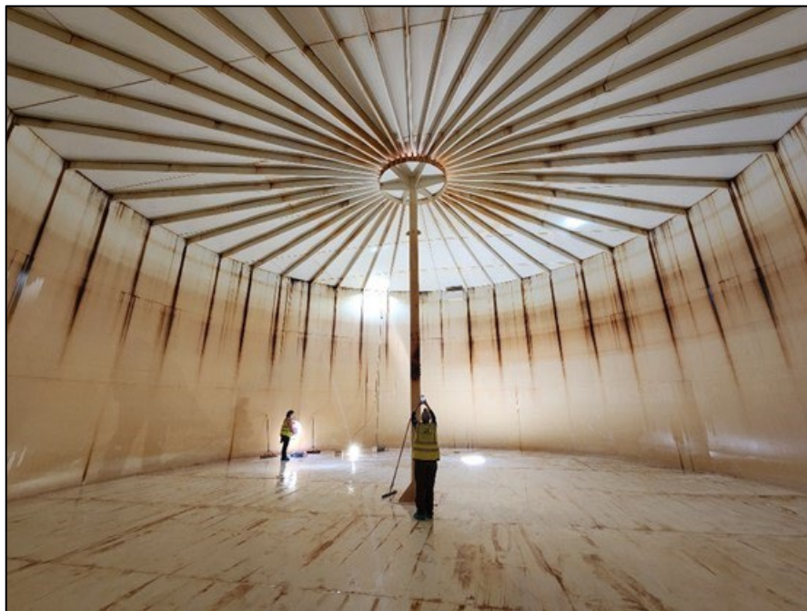
Cordillera West Tank 1 interior inspection
