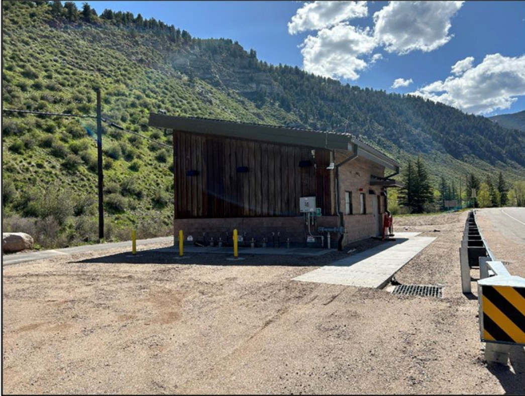
Exterior view of completed lift station
