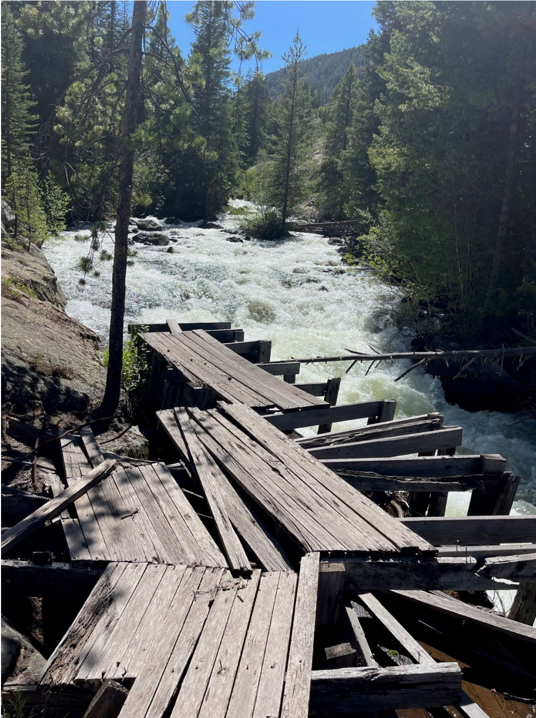
Photograph of Bolts Ditch diversion structure
