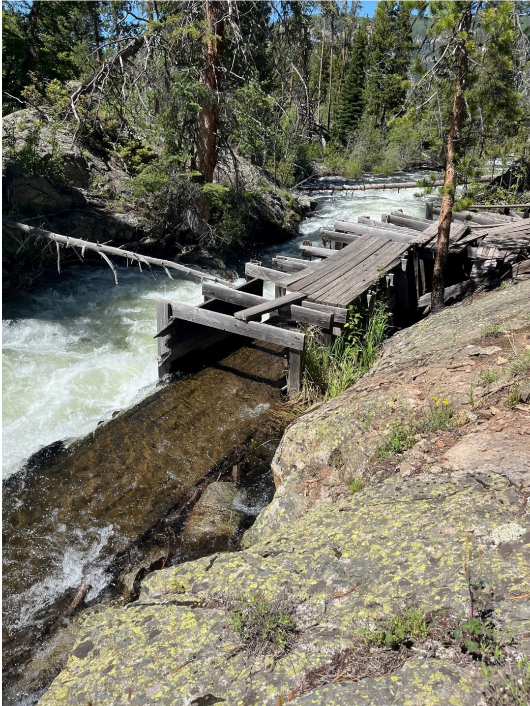
Photograph of Bolts Ditch intake and diversion structure
