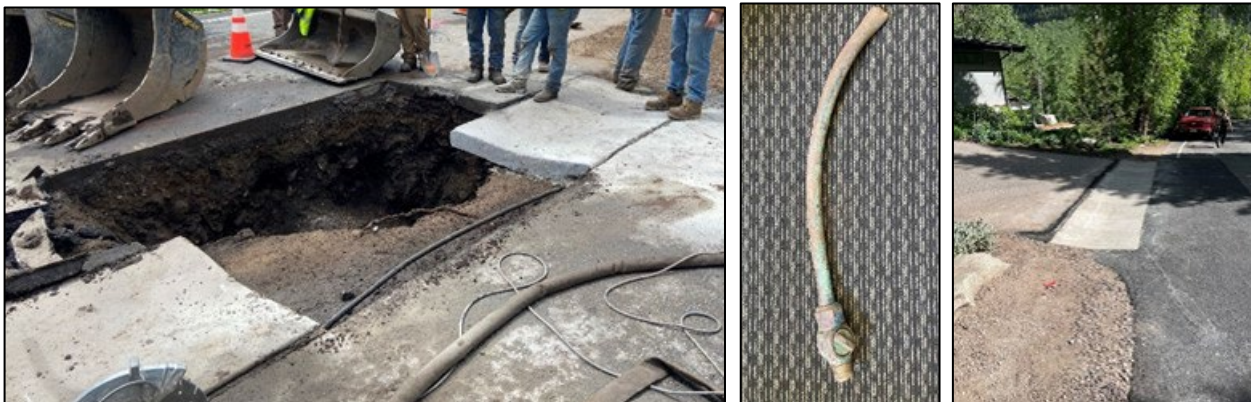
East Vail water main repair (excavation left; damaged service center, completed repair right)
