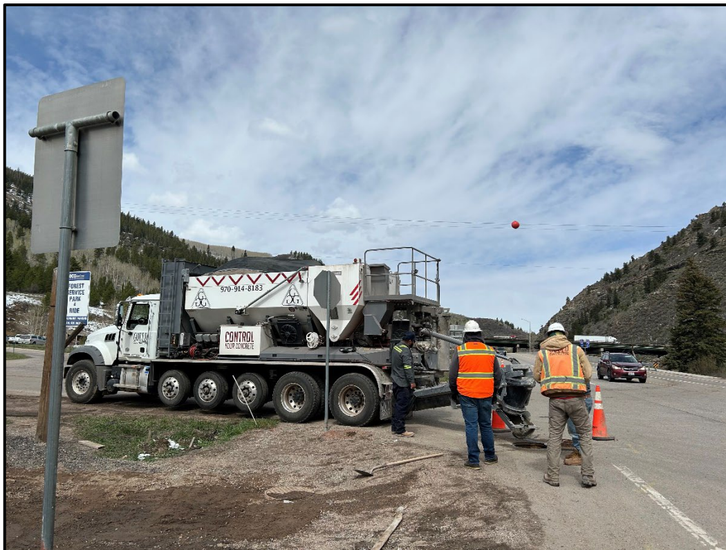
Abandonment of manholes in the old gravity sewer line
