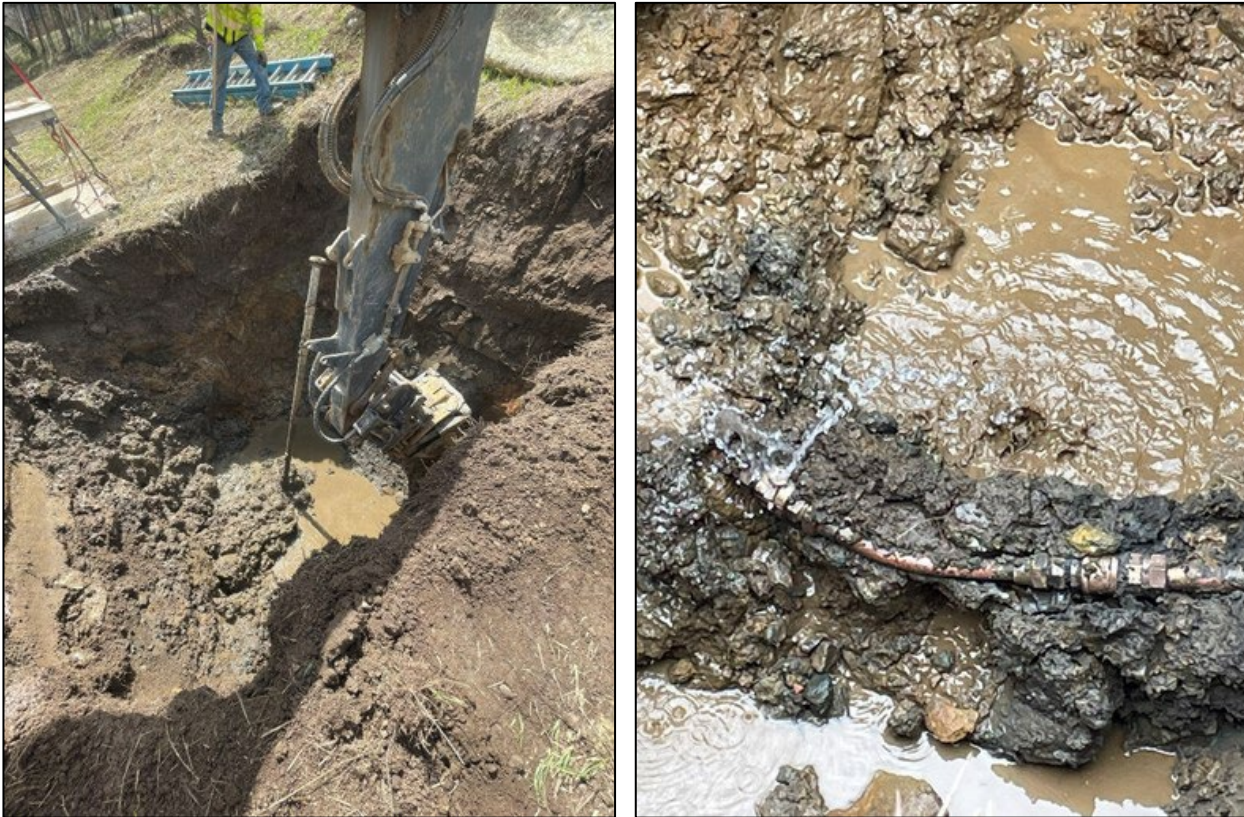
Curb stop repair (excavation left; leaking valve right)
