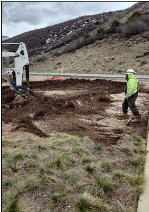
Site preparation for Wildridge Tank 1 waterproofing
