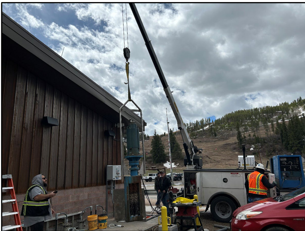
Installation of bail to lift grinder for maintenance
