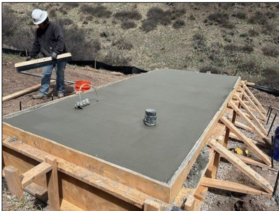
New concrete pad for the generator at Wildridge BPS 1
